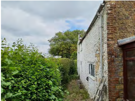
Figure 22: The residential building's western elevation and hedgerow forming the Site's boundary
