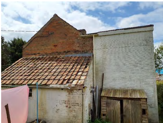
Figure 30: Loose and missing tiles
