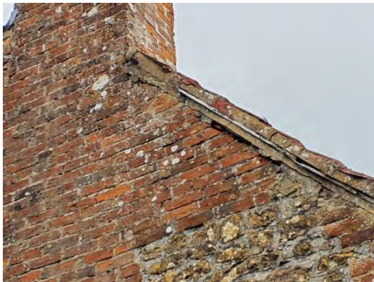
Figure 30: Loose and missing tiles
