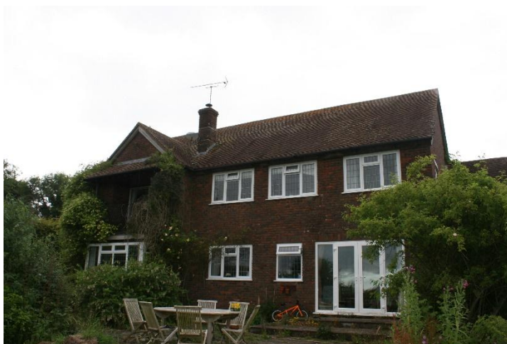
Photo 8: South elevation of the house (B1).
