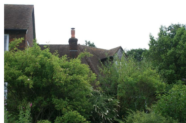
Photo 9: South elevation of the annexe (B1).
