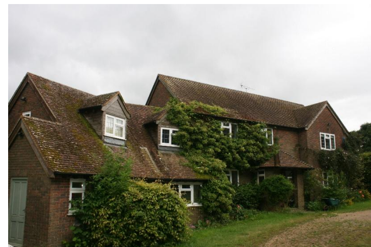
Photo 12: Northeast view of the house (B1).
