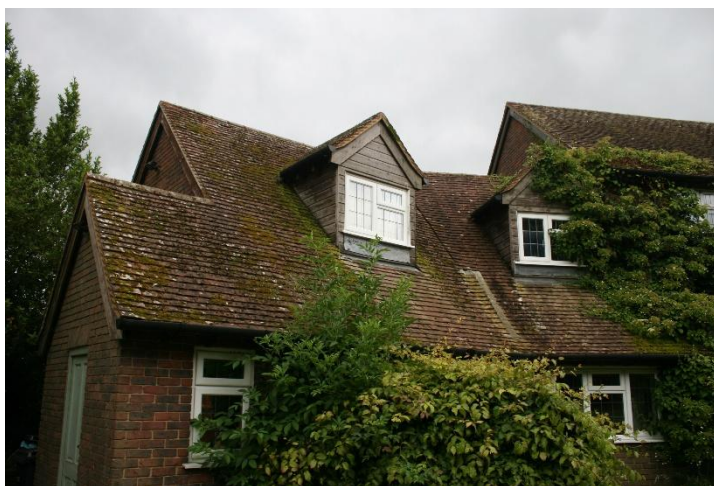
Photo 11: North elevation of the annexe (B1).
