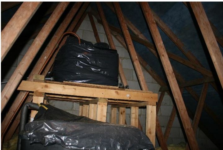
Photo 1: Water tank in the loft void.
