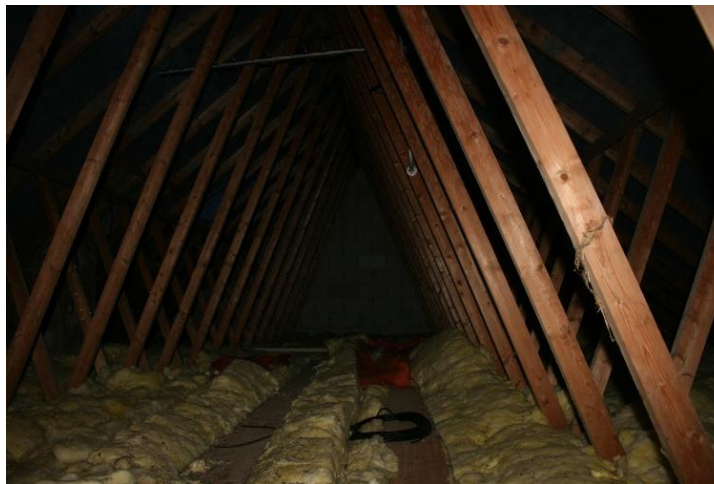
Photo 2: Inside the loft void.
