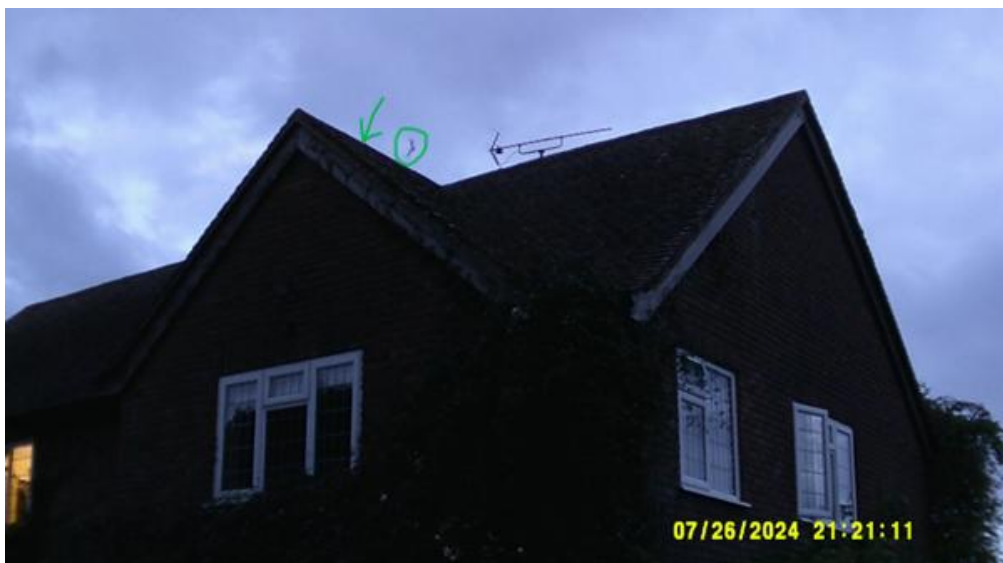
Figure 2: Common pipistrelle exit point on the northwest gable ridge.
