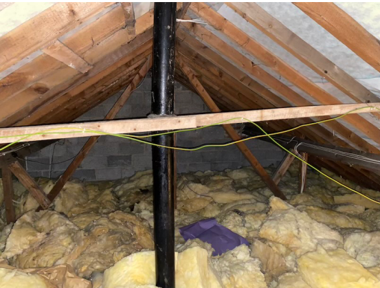
Plate 3 - Internal Roof Void
