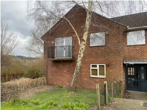
Plate 2 –East Gable of Eastern Building
