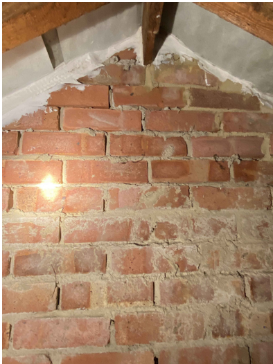
Plate 4: Filled Gable Walls and Internal Roof Void Walls
