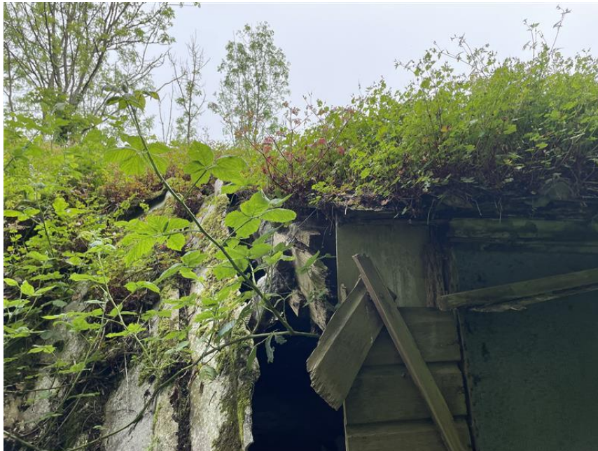
Photograph 10: Ivy cladding on B1
