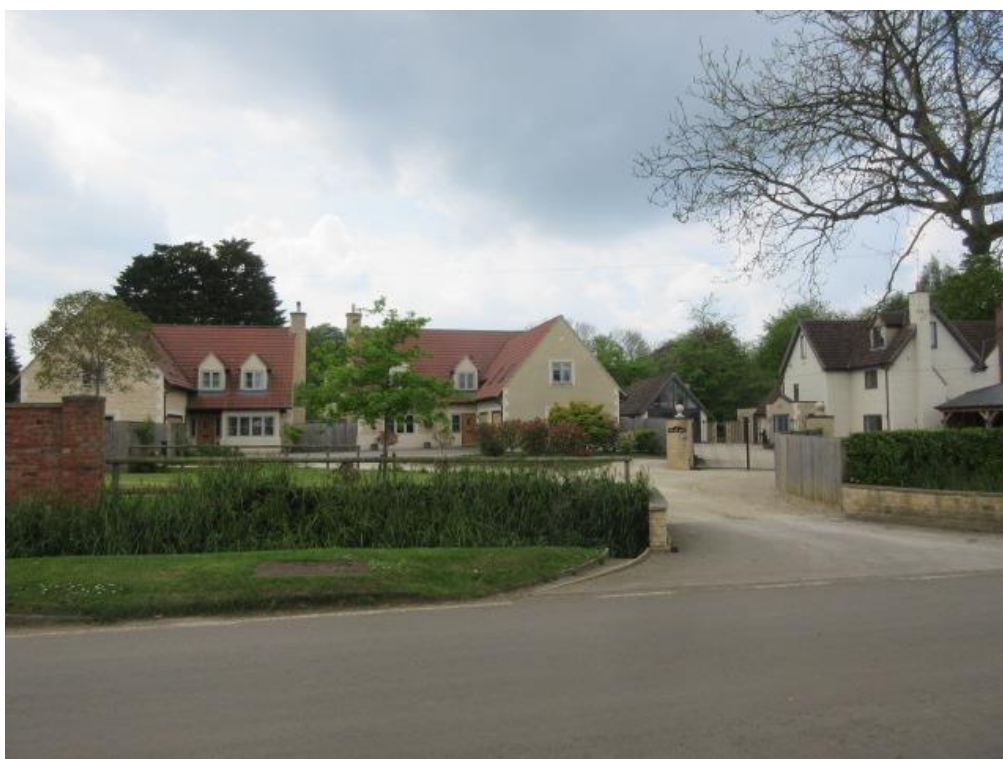
Plate 16: New development east of site at junction, looking west
