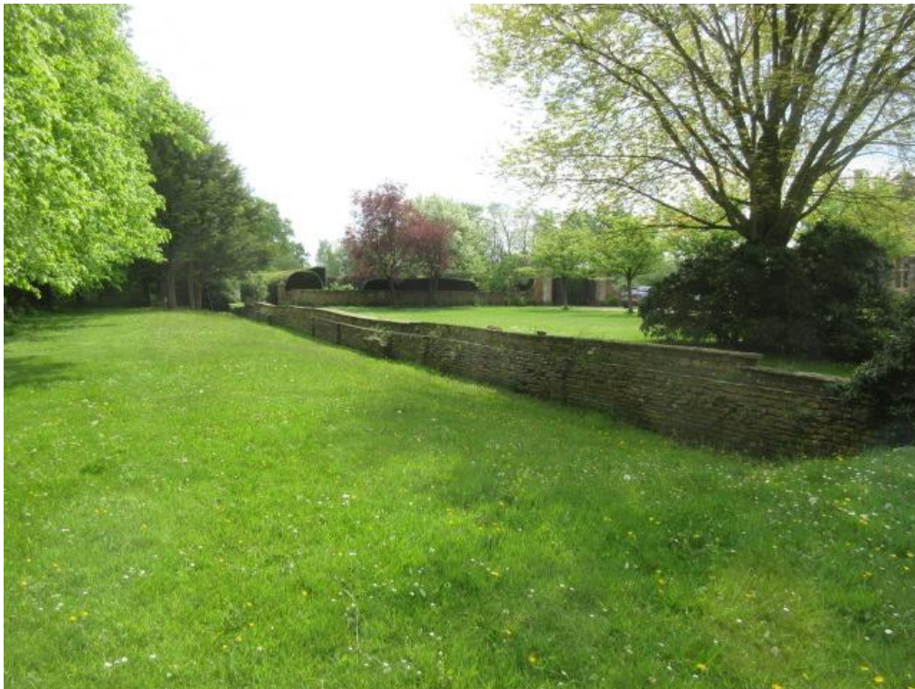
Plate 14: Ha-ha defining formal gardens at Seagry House, looking west
