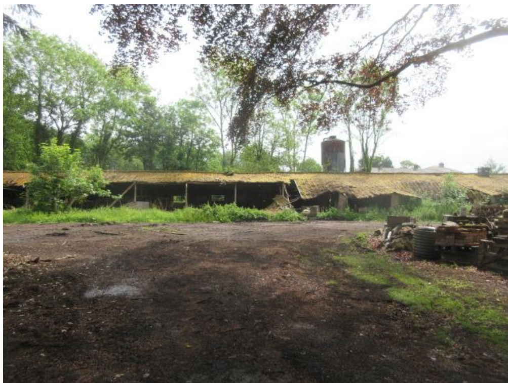
Plate 8: Large existing warehouse within site, looking south east
