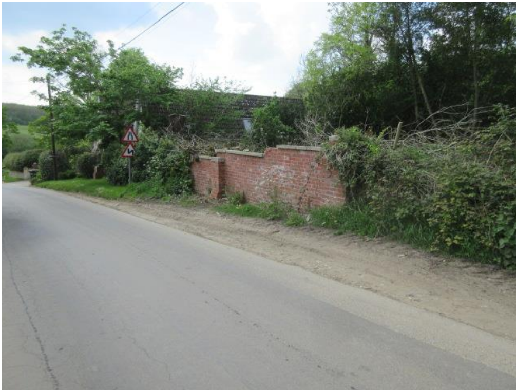
Plate 11: Existing brick wall adjacent to Henn Lane, looking west
