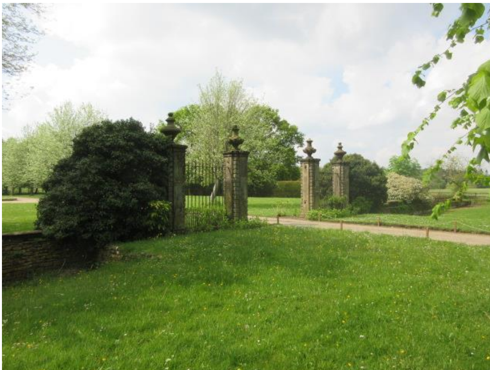
Plate 2: Main entrance gatepiers, railings and gates north east of Seagry House, looking north west
