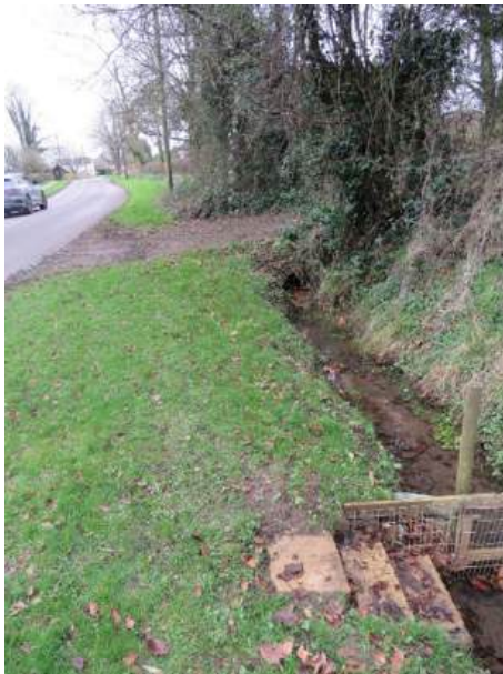
Drainage Ditch on West Side of Startley Road
