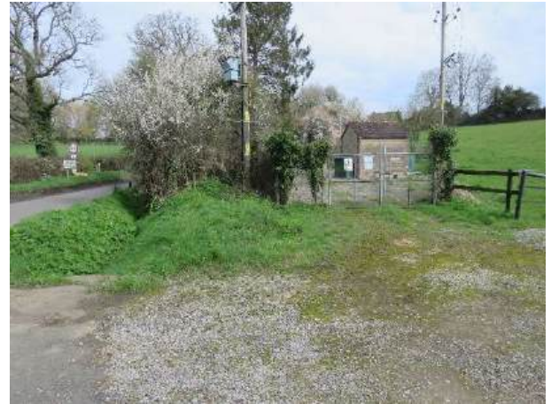
WW Foul Pumping Station on East Side of Henn Lane
