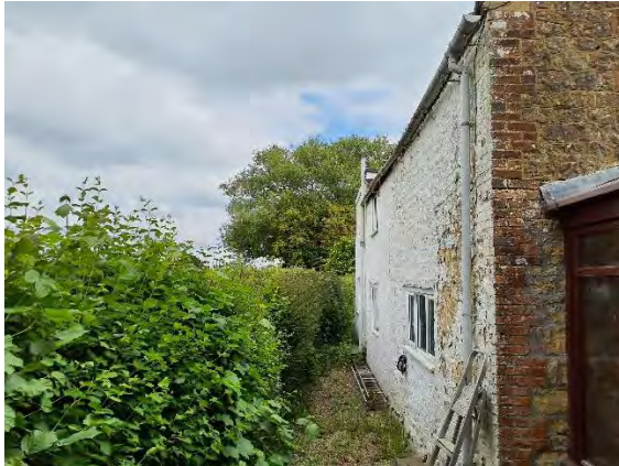
Figure 10: The residential building's southern elevation from the east side along with the non-native and ornamental hedgerow
