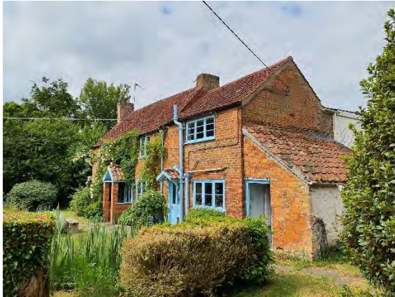
Figure 14: The residential building's eastern and northern elevation
