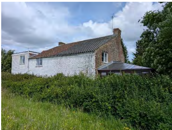
Figure 12: The residential building's western and southern elevation
