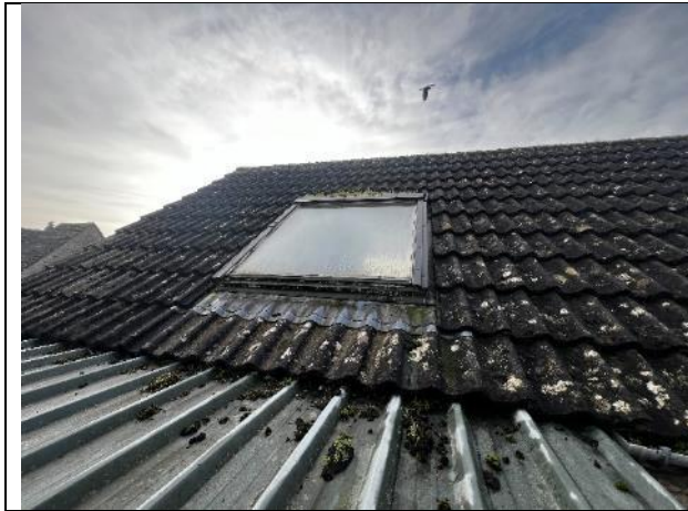
Figure 19: Intact roof tiles on B3
