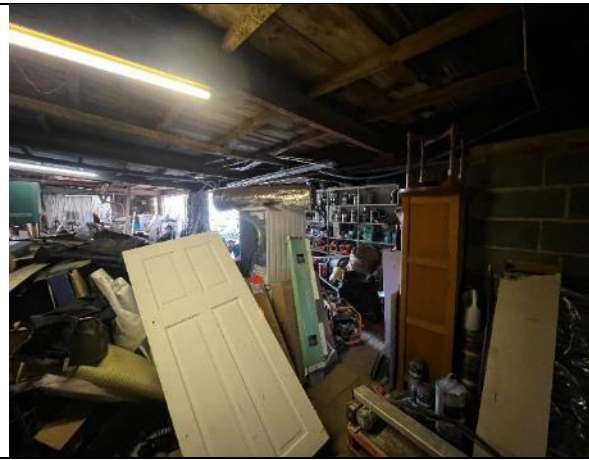
Figure 17: Interior of B2
