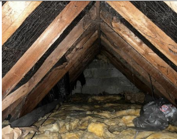
Figure 8: Internal loft void, looking south
