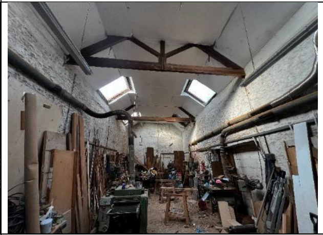
Figure 18: Interior of B3
