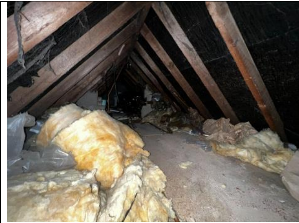
Figure 7: Internal loft void, looking north
