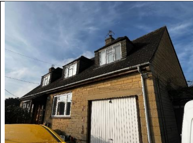
Figure 1: East and north elevations of B1
