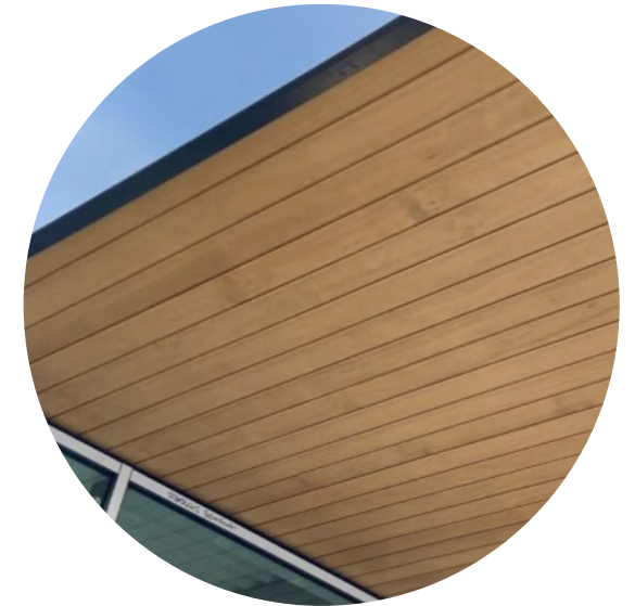
Cedraal cladding to soffits and plant screens
