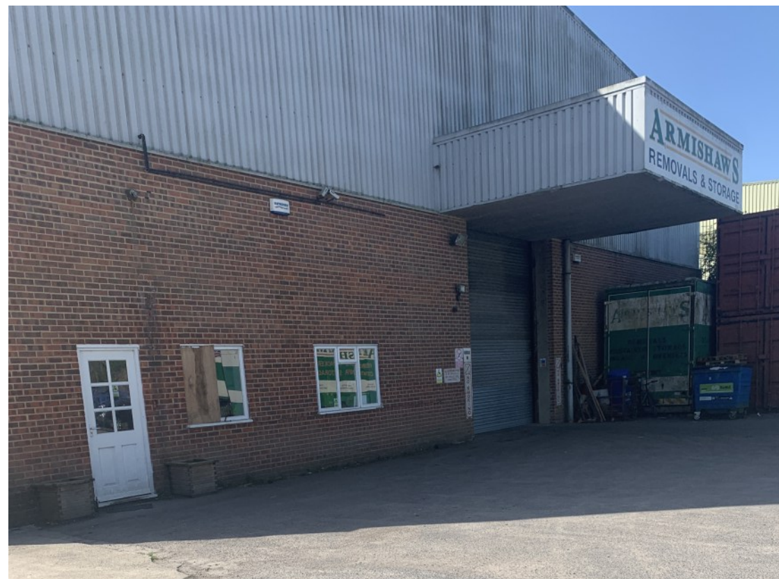
Existing Armishaw's entrance to be amended
