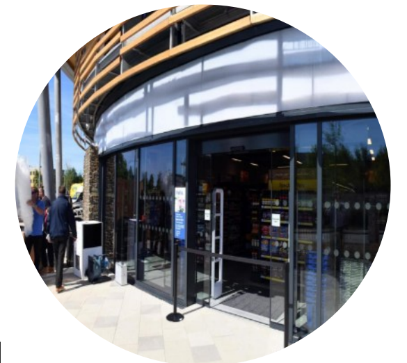
Example of shopfront glazing and brise soleil
