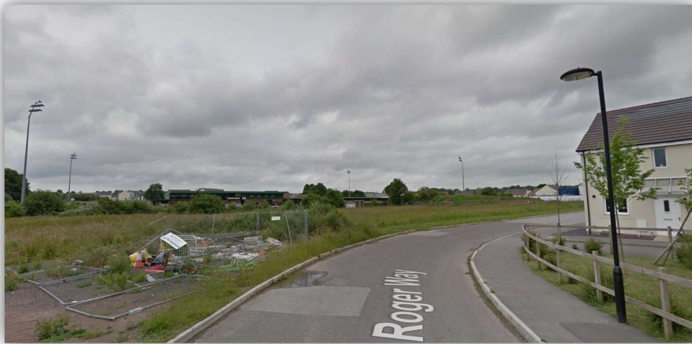
Figure 3.3: Existing street lighting columns
