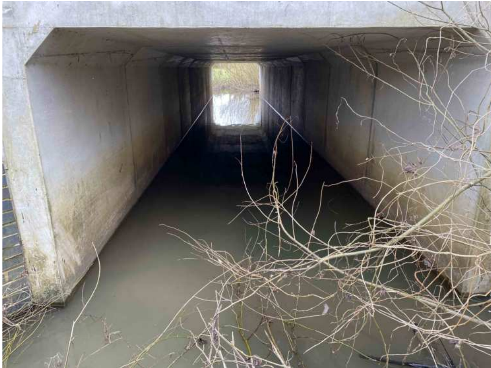
Figure 23: Gregor Drive Culvert Entrance
