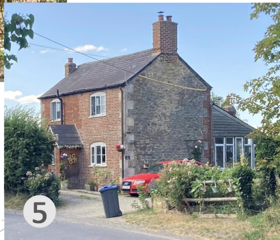
Image 5. (no.2 Main Street) Casement joinery with arched brick lintels, warm brickwork, stone quoins under a gabled slate-covered roof form.
