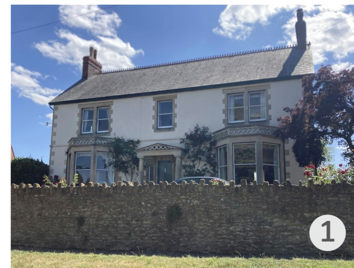
Image 1. no.5 Main Street is a key influence by virtue of its symmetrical principal elevation, ground floor bay windows, dressed stone quoins, sash joinery, stone window sills & lintels, slate roof covering, chimney details and roof gables with painted wood bargeboards.
