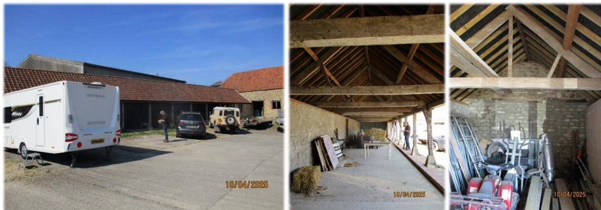
Building 2 exterior and interior
