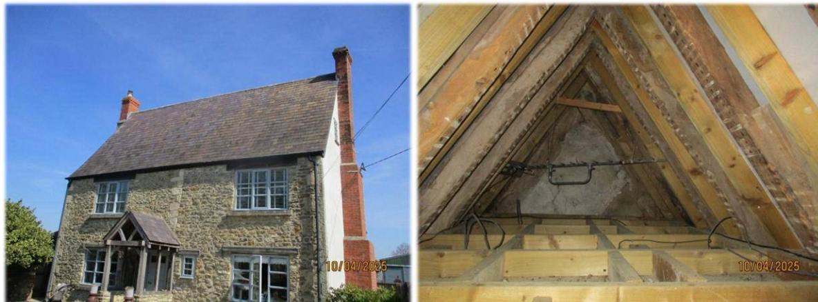
Building 1 exterior and sealed attic
