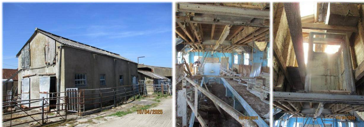
Building 4 exterior and interior
