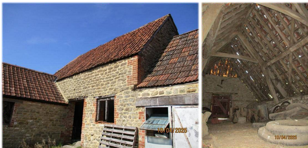
Building 3 exterior and first floor hayloft
