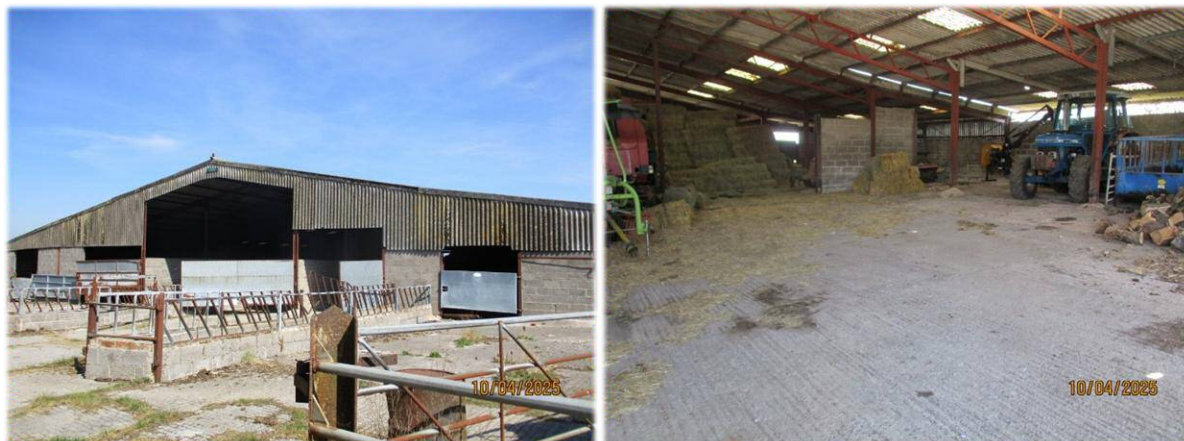
Building 7 exterior and interior
