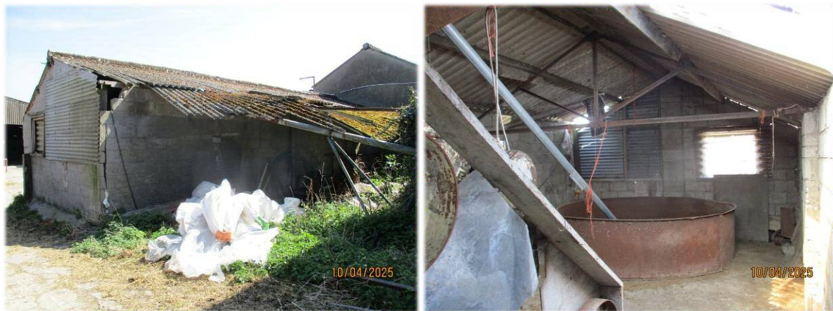
Building 9 exterior and interior
