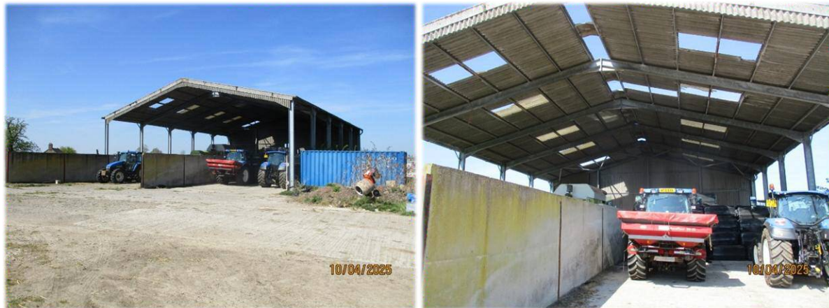
Building 12 exterior and interior
