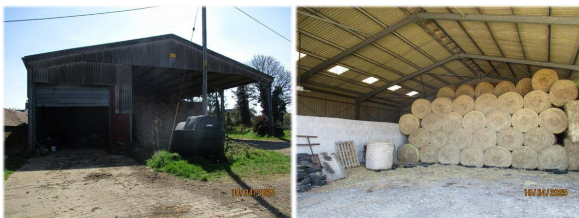
Building 11 exterior and interior
