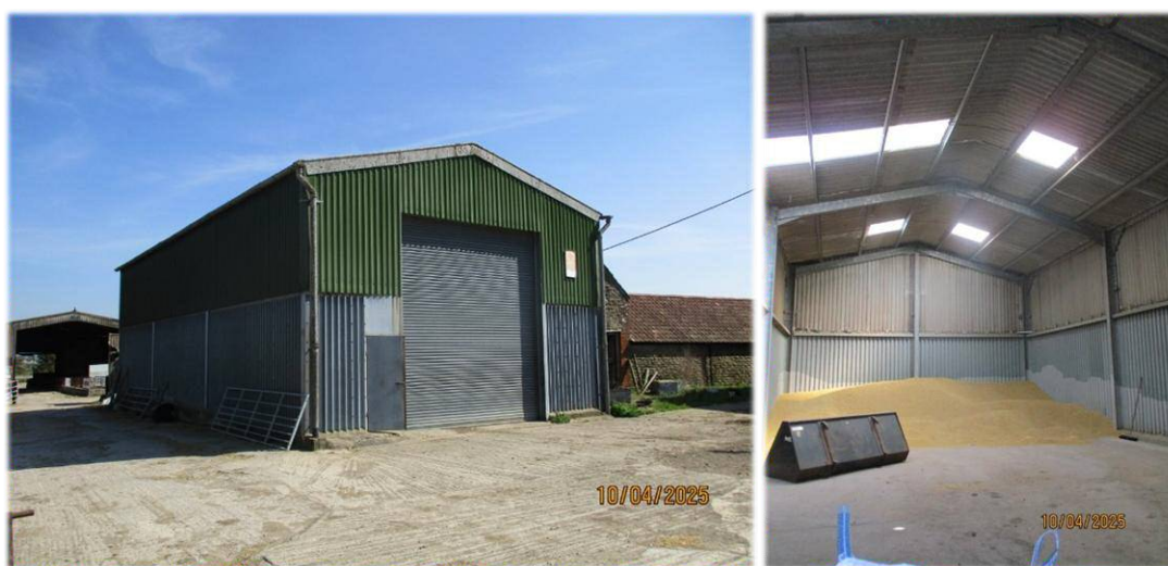
Building 10 exterior and interior
