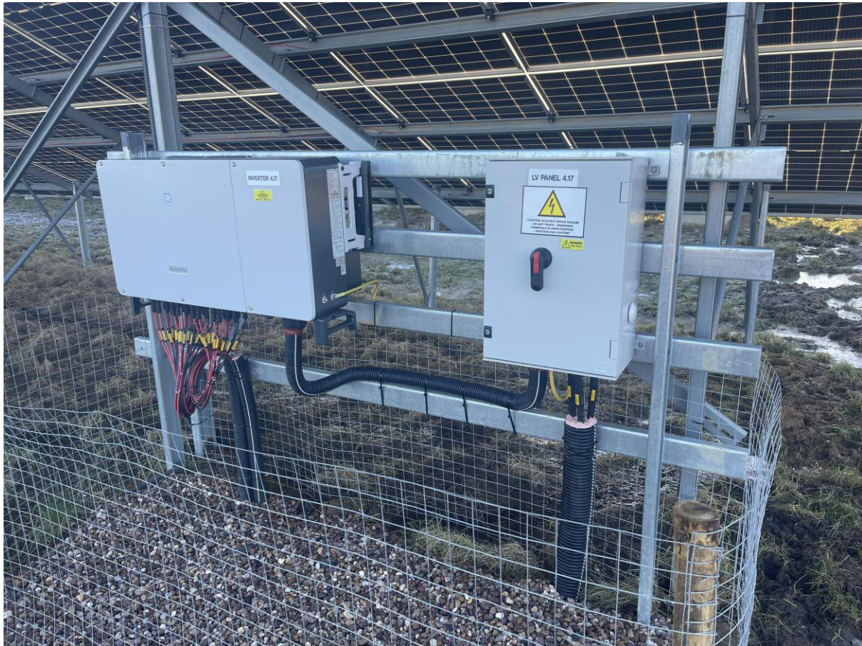
Figure 5-2: Example of string inverter
