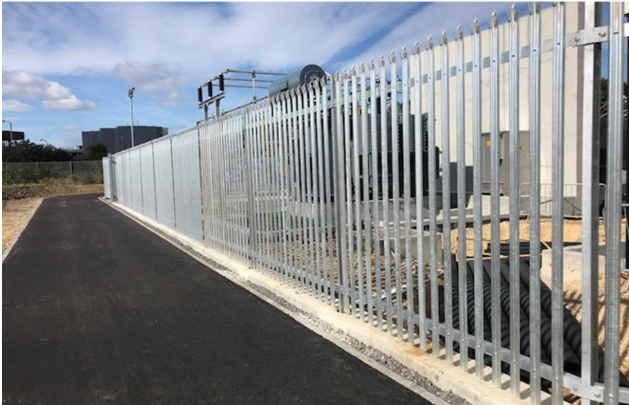
Figure 5-5: Example of palisade fencing to enclose substation compound
