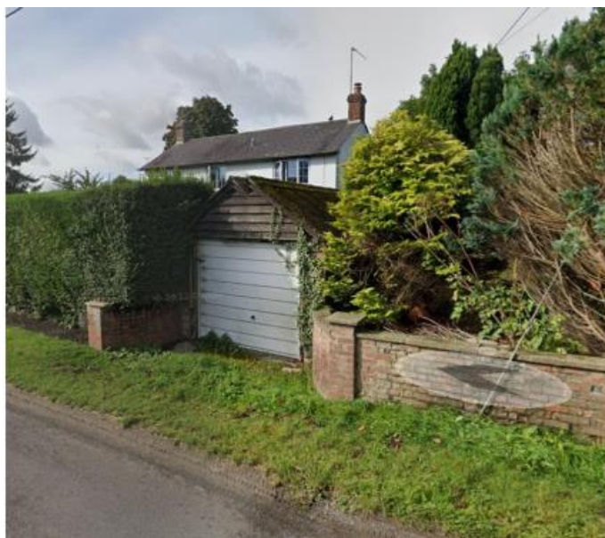
Fig. 6: View of the existing garage, looking south-west from The Street, with Iris Cottage beyond.
