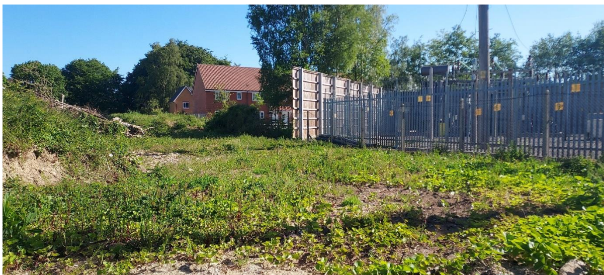
Photo 2: The south-east corner next to the electrical substation with an earth pile to the left
