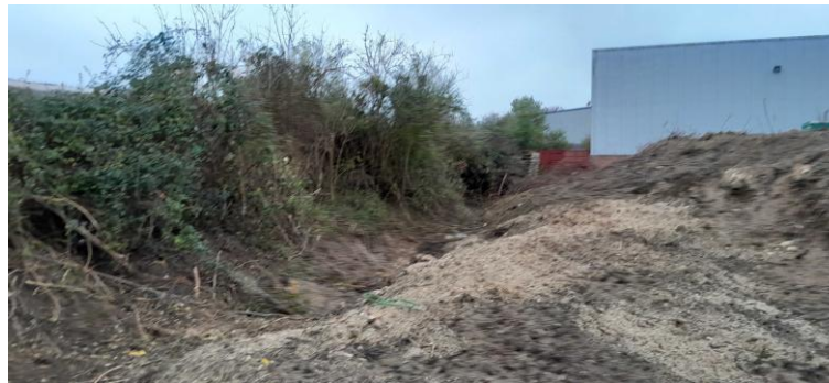
Figure 5 - View of hedgerow to the south of the site showing excavations where vegetation has been dragged away using machinery.
