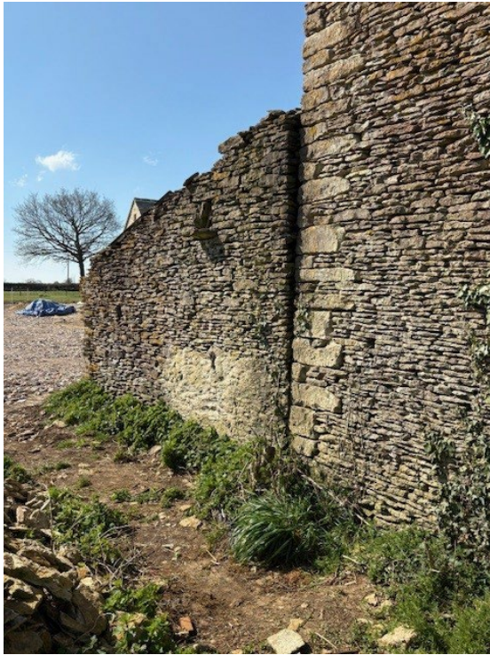
PLATE 17 -- UNBONDED WING WALL
