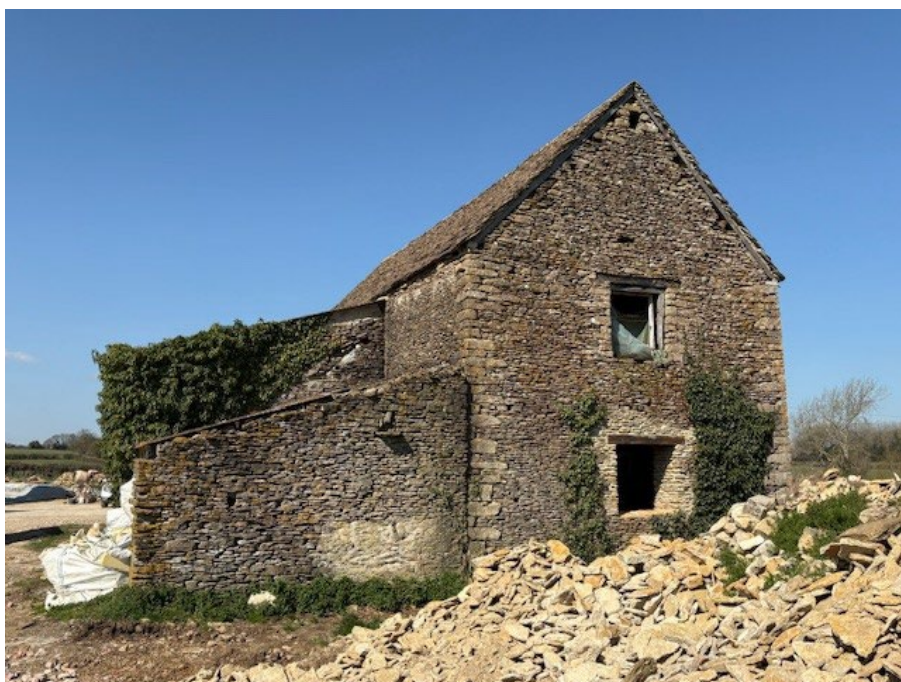
PLATE 09 -- TIMBER LINTELS OVER OPENINGS
