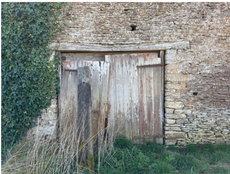
PLATE 14 -- BADLEY DEFLECTED TIMBER LINTEL
