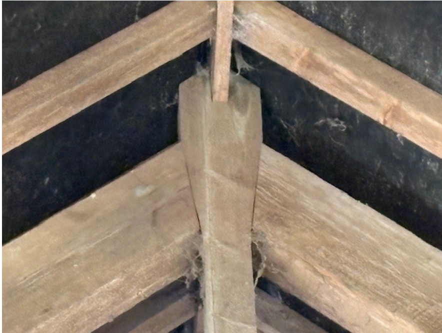
PLATE 07 -- TIGHT TRUSS JOINT AND RIDGE
