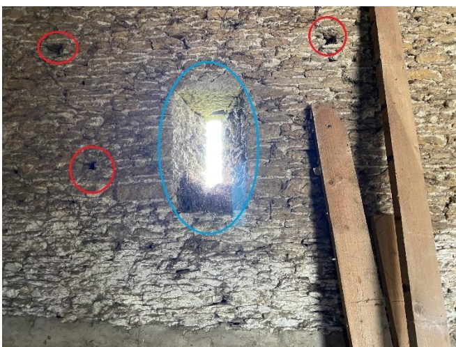
Photograph 5: Internal features on northern wall.
