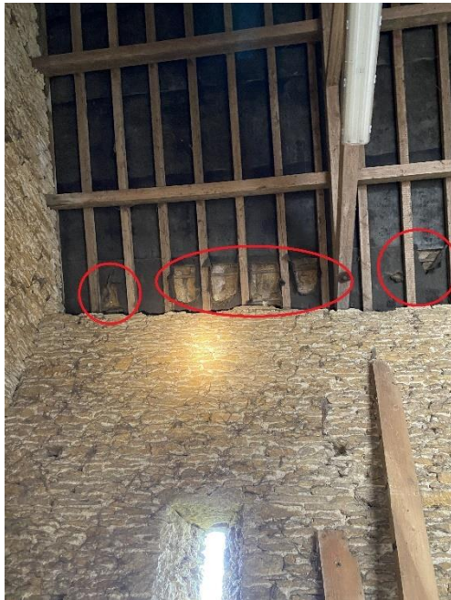
Photograph 7: Internal roof PRFs.
