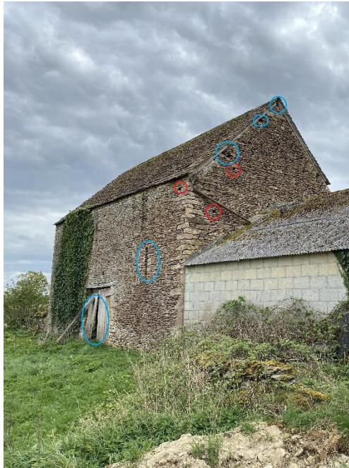
Photograph 3: Northern side of the building.
