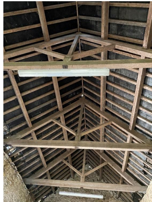
Photograph 8: Internal wooden beams.
