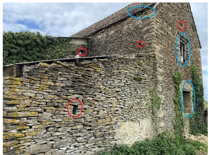
Photograph 2: Eastern side of the building.
