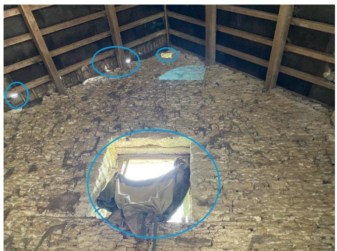
Photograph 6: Internal access points eastern wall.
