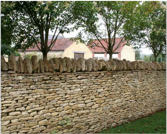
Image 1: Local coursed walling style (image supplied by Landscape Officer at Wiltshire Council)
