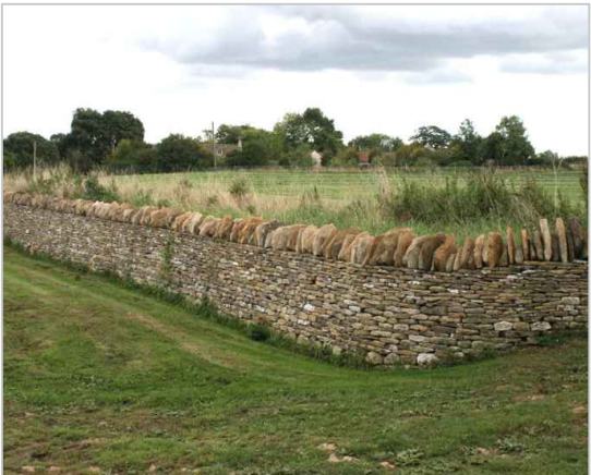
Image 2: Local coursed walling style (image supplied by Landscape Officer at Wiltshire Council)
