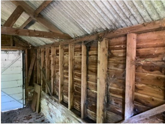
3: Timber weatherboard wall over brick base.
