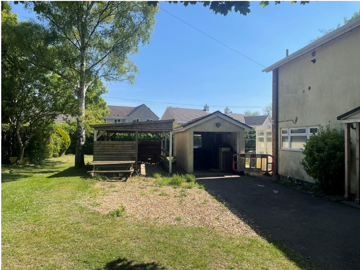
Photograph 1: showing a view of the site
