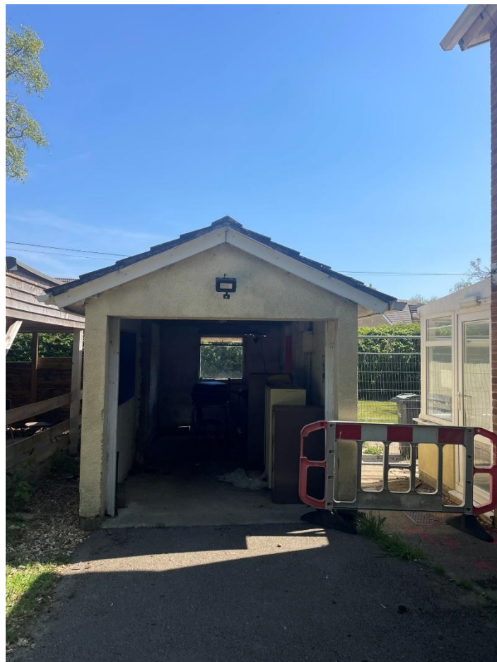
Photograph 5: showing a view of the inside of Building 2 (looking south)
