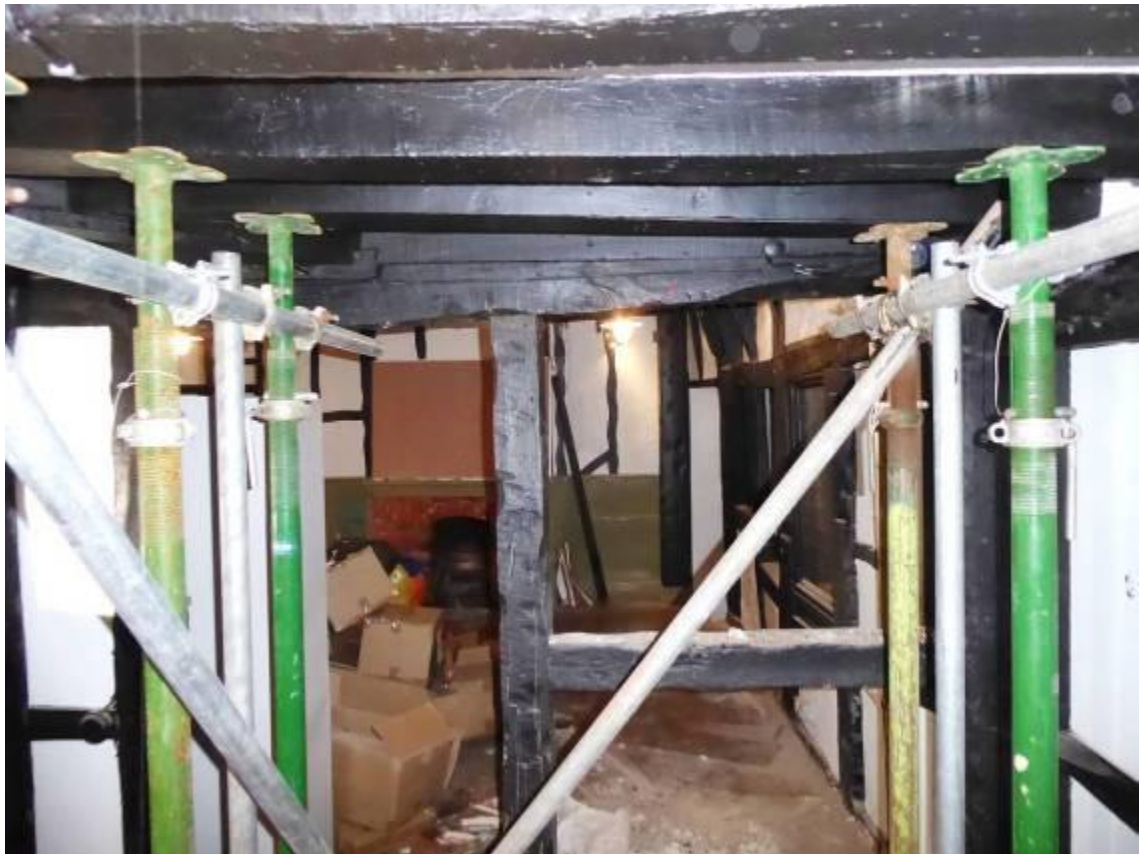
Fig 3.2.3: Propping at ground floor level
