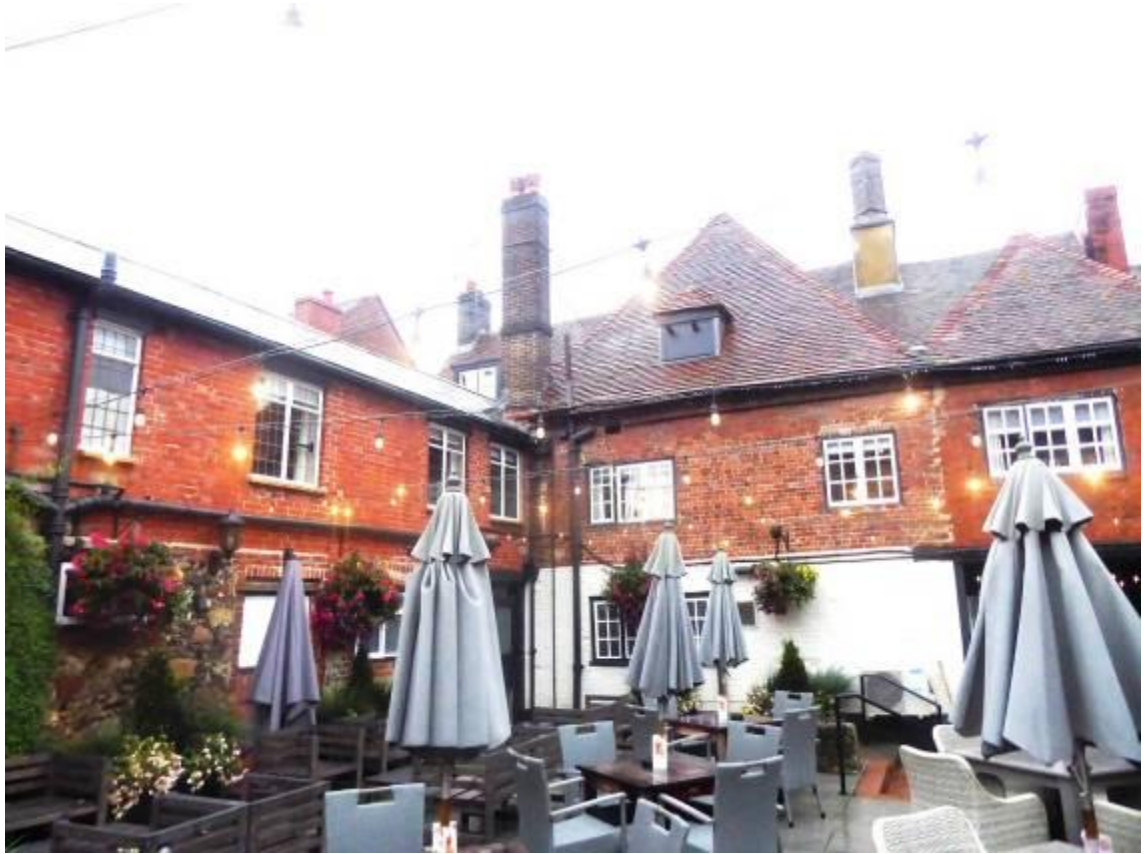
Fig 4.1.7: Rear east wing (east)
