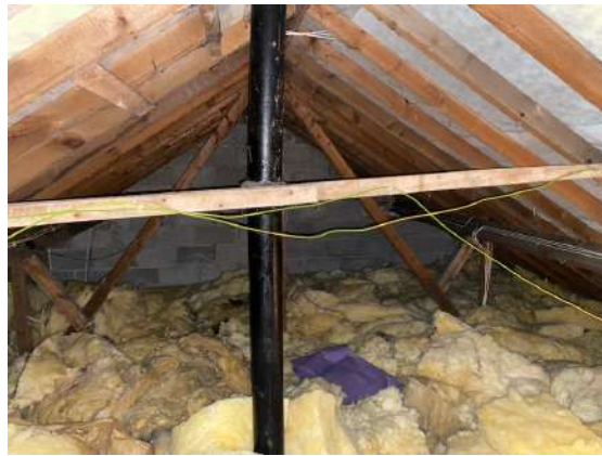
Plate 14: Internal Roof Void
