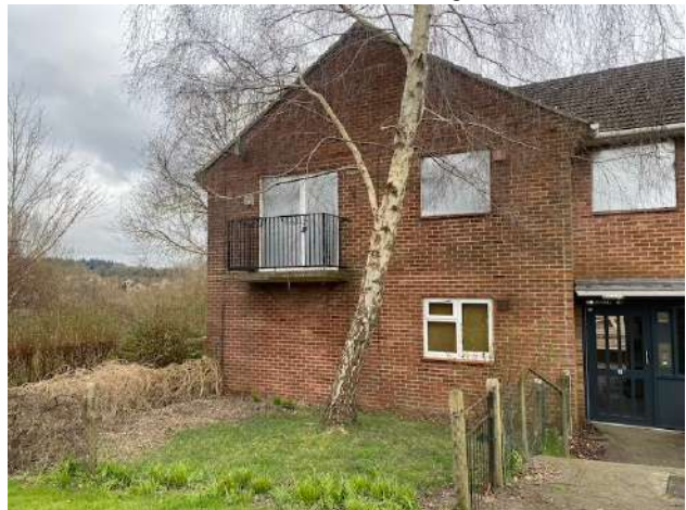
Plate 12: East Gable of Eastern Building
