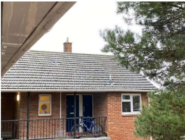
Plate 11: 48-60 Alcock Crest Roof Aspect
