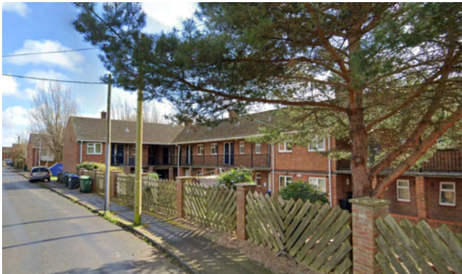
FIG 03: View Towards 43-60 Alcock Crest
