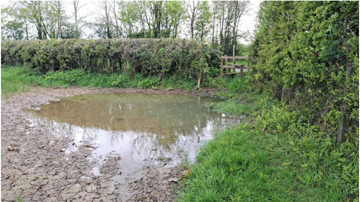
Photo 1 ponding in north-western corner of site adjacent to public footpath
