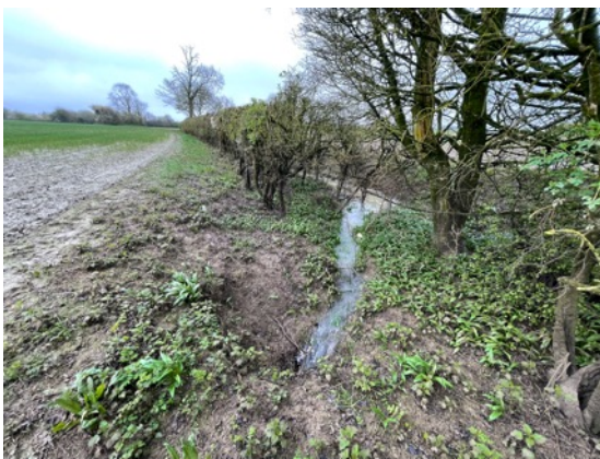
5: End of flowing wet ditch along the south west boundary.
