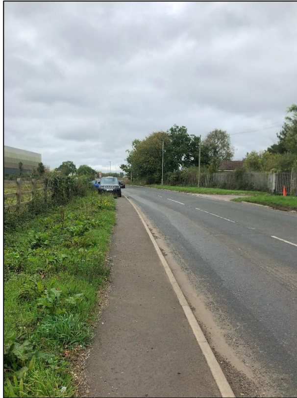
Photograph 1: B4122 Existing Conditions
