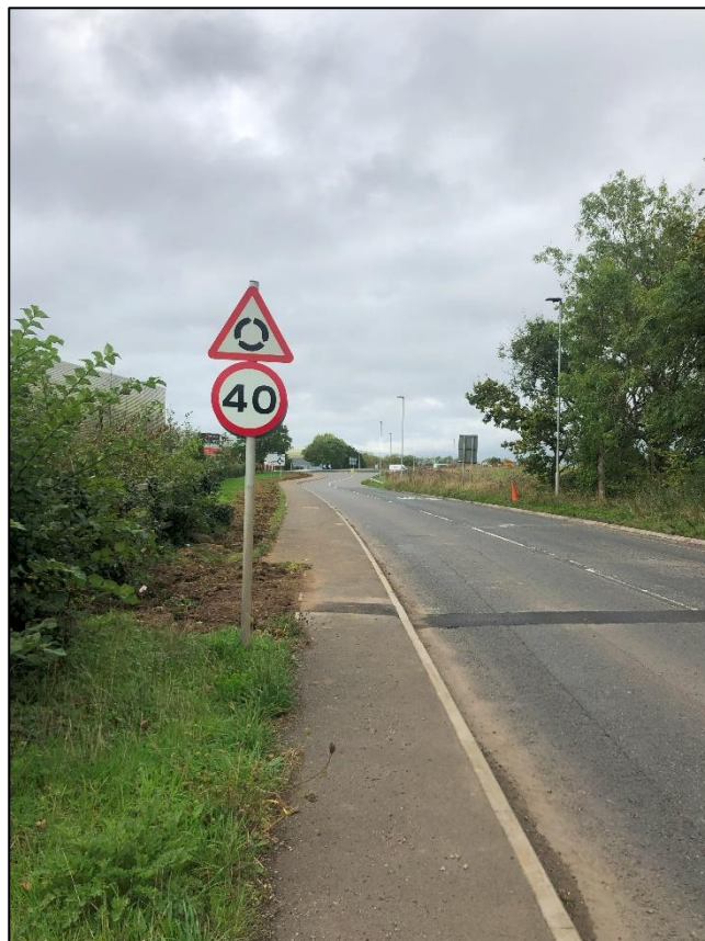
Photograph 2: B4122 Existing Footpath Conditions
