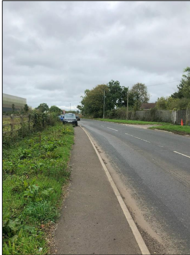
Photograph 1: B4122 Existing Conditions
