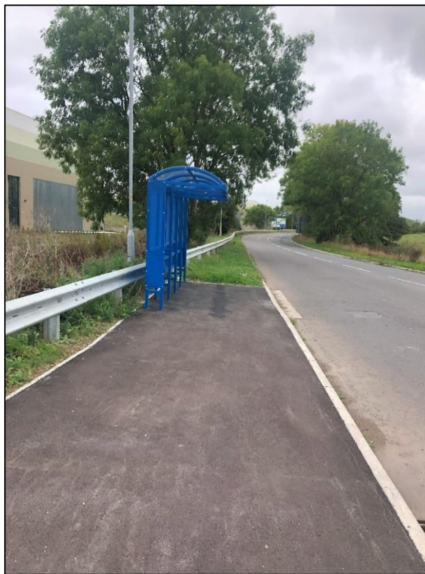
Photograph 3: Bus Stop Conditions
