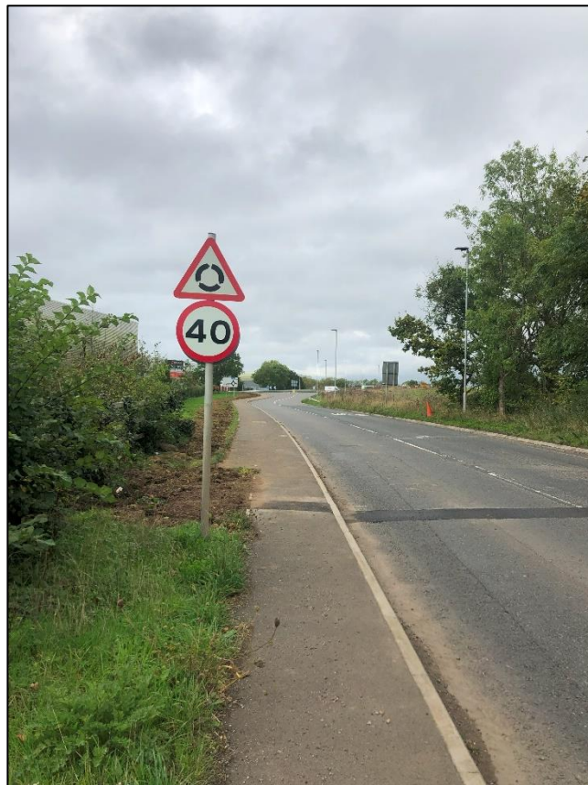
Photograph 2: B4122 Existing Footpath Conditions
