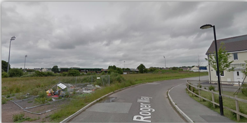
Figure 3.3: Existing street lighting columns
