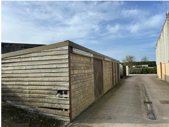
Lock up units associated with Unit12
