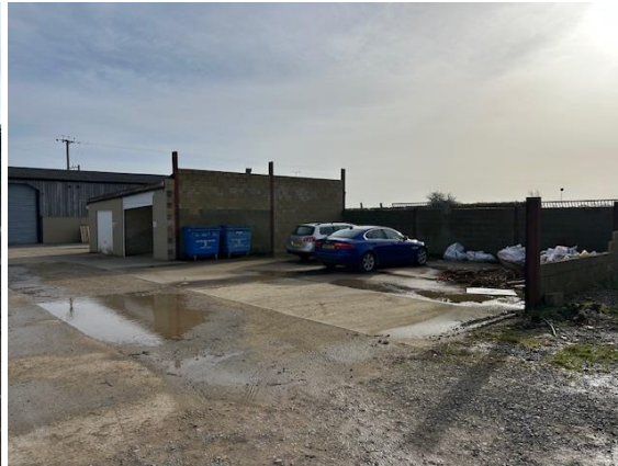
Open yard west of Units 10 and 11
