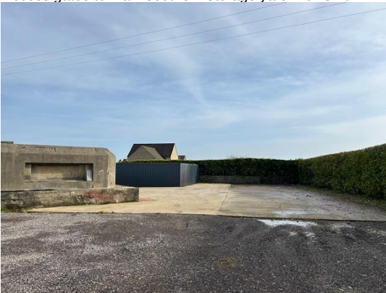
Unit 12 set within the vacant yard, bar the containers beyond.
