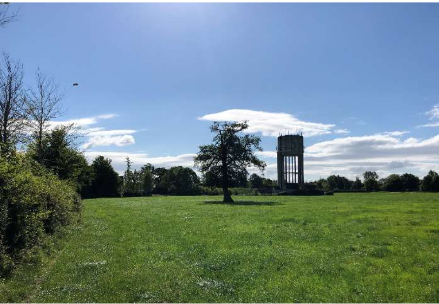
Photograph 5 – Looking east, showing open fields with the water tower and infrastructure situated to the east.
