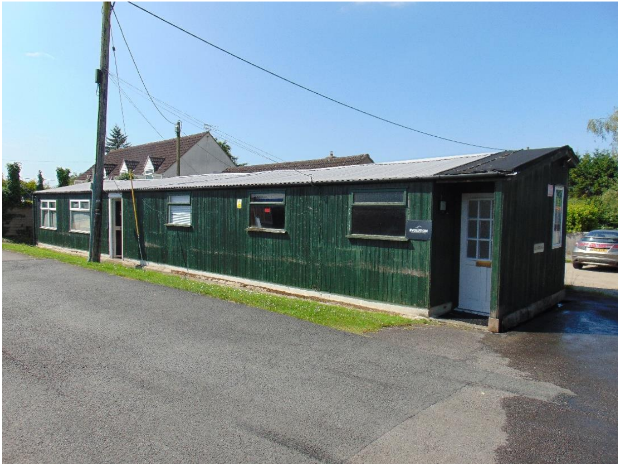
Photograph 5: showing the northern and eastern elevations of Building 2
