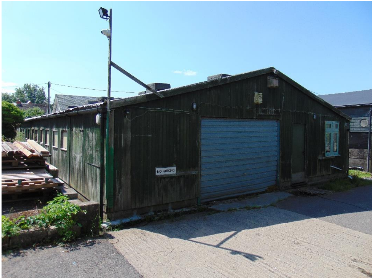
Photograph 7: showing the northern and eastern elevations of Building 4
