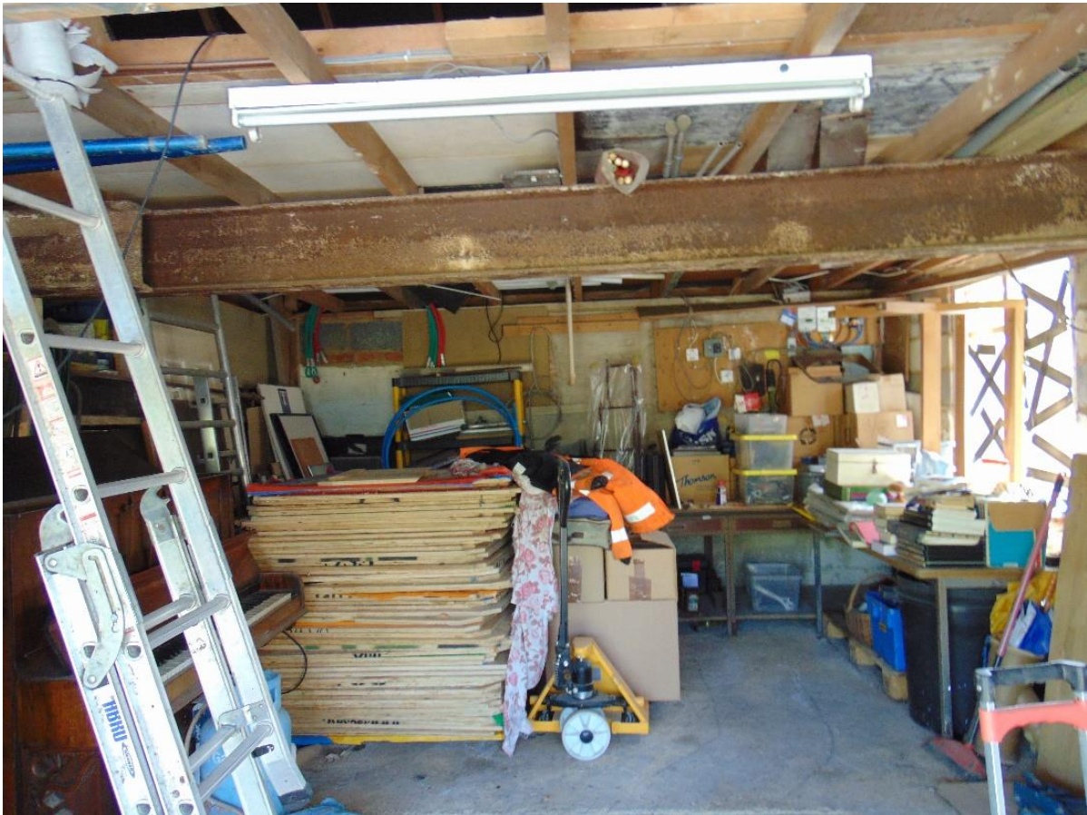
Photograph 5: showing the interior of Building 1
