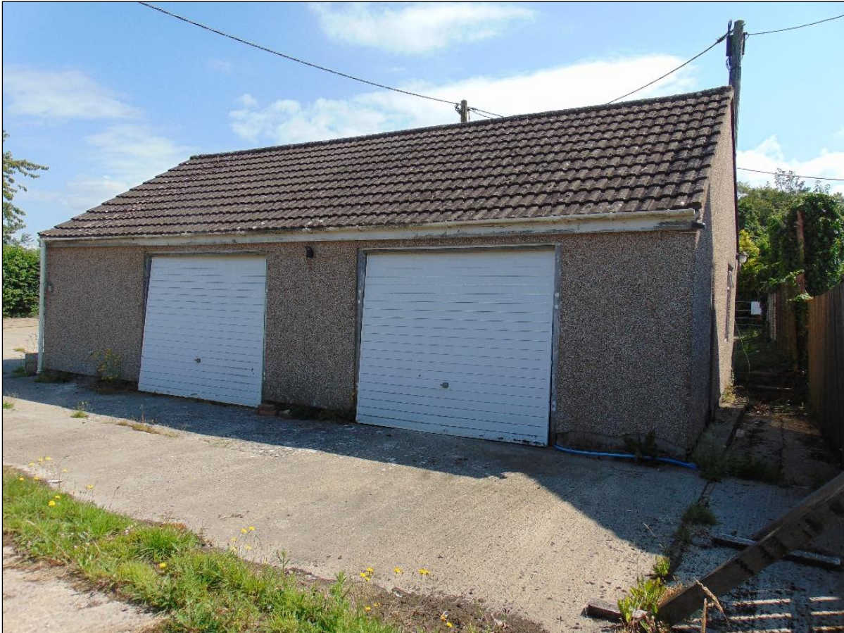
Photograph 5: showing the western elevation of Building 1
