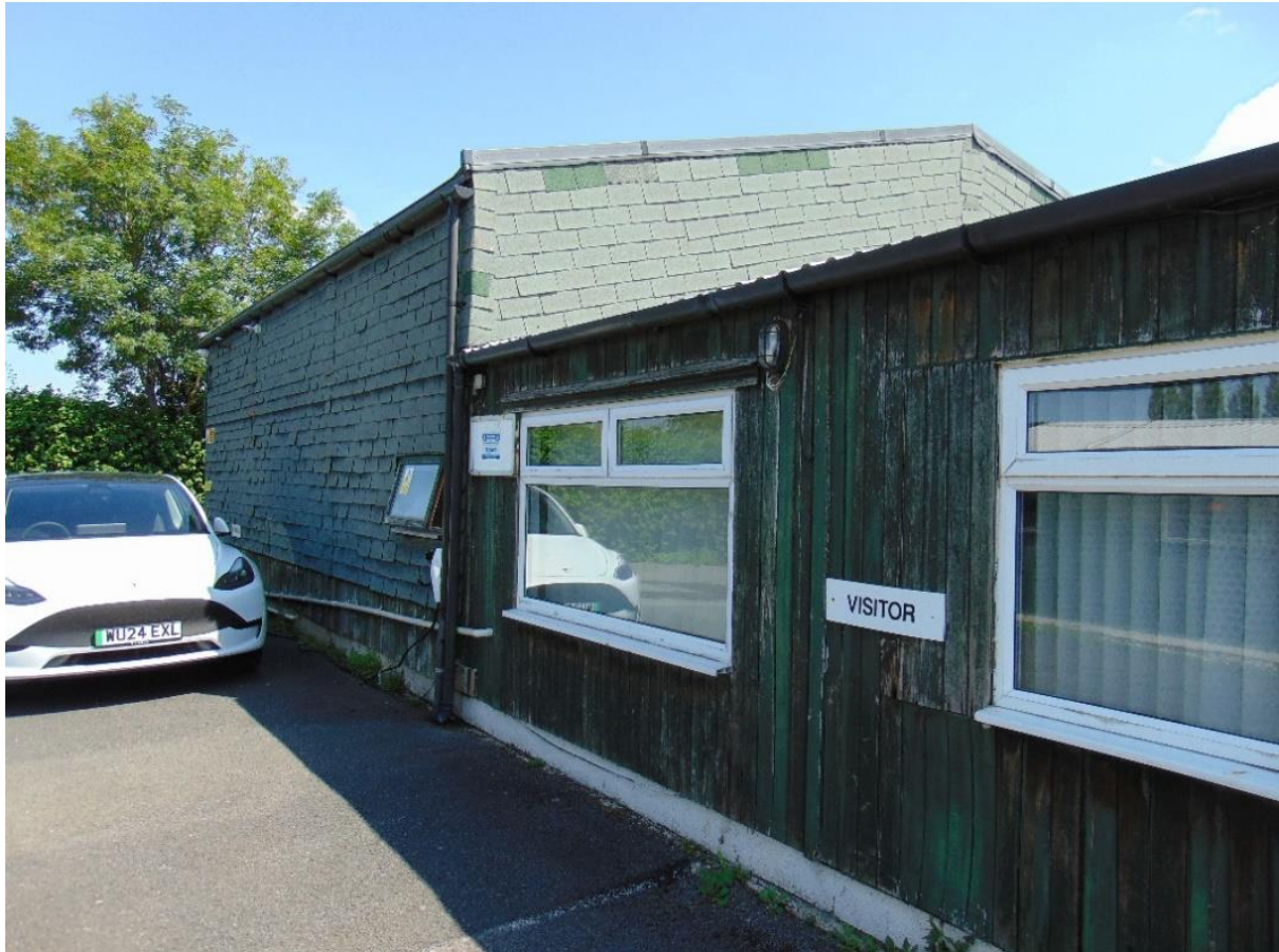
Photograph 6: showing the western elevation of Building 3 (looking north)
