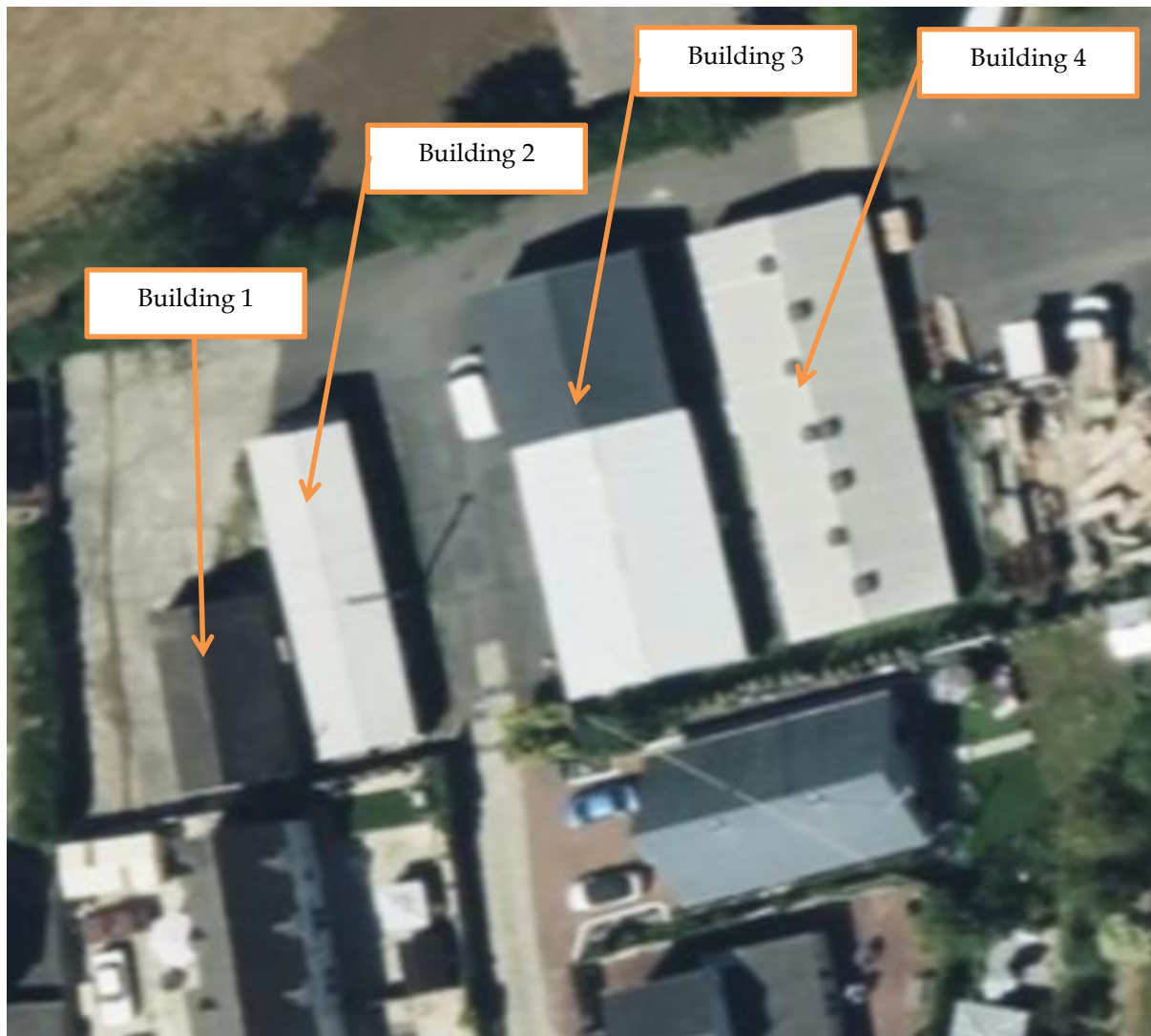
Figure 2: showing the buildings on site
