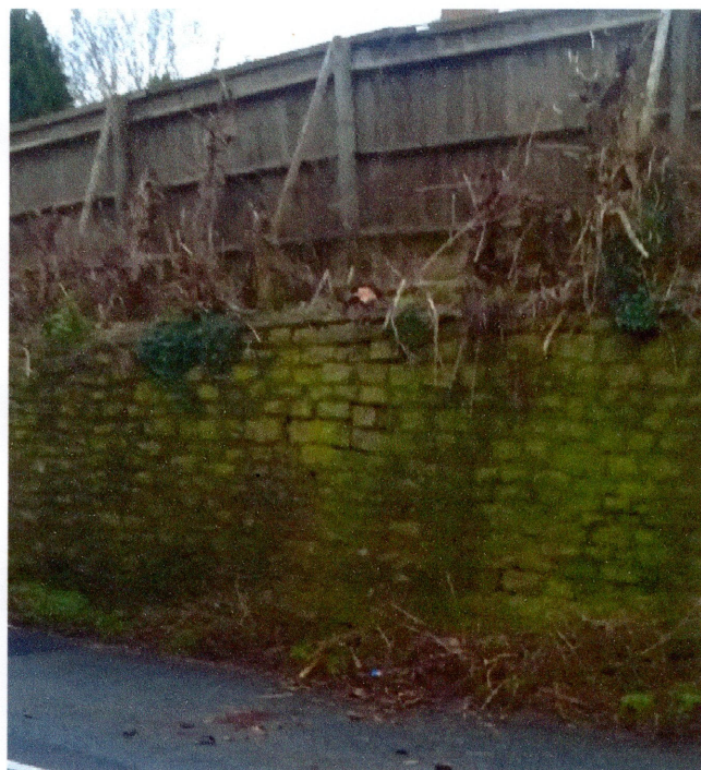
Above Right. Side effect on road with severe camber. The top of a large vehicle can lean up to 25cm (approx 10inches). Drivers need to 'choose position' to ensure it will not collide with buildings, other vehicles or street furniture. NOTE you can see from the end of trunk that the tree was alive. The road is too narrow for driver to choose position of lorry therefore has to cause damage. SOURCE Safediving for Life, partner of DVSA.
