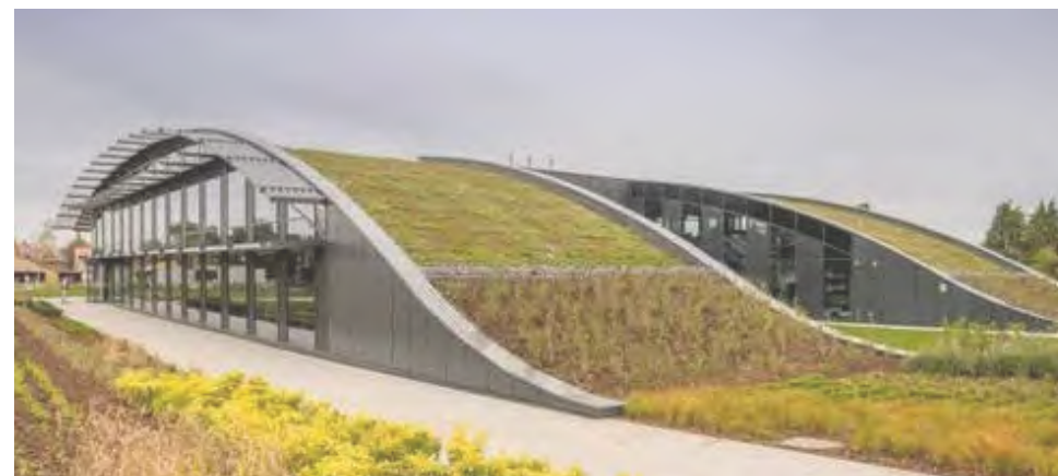
Roof - Sensible Architecture
