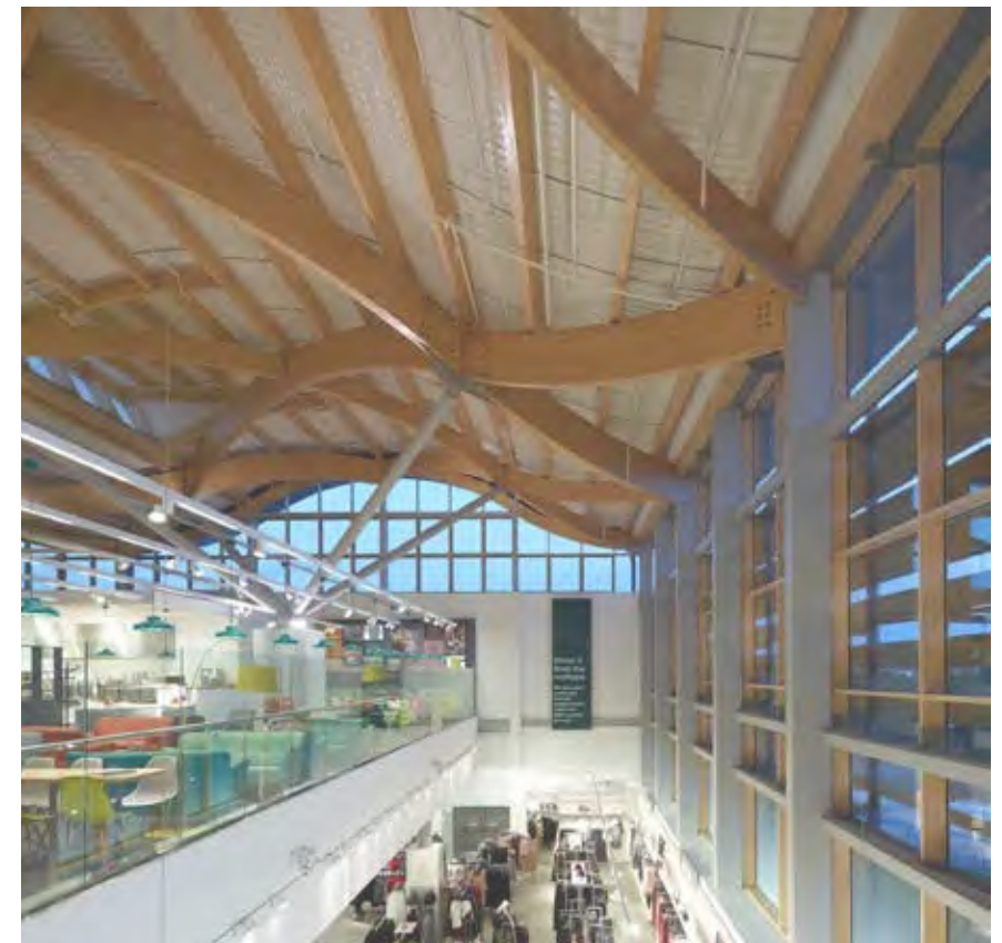
Sustainable Material - Exposed Glulam Structure
