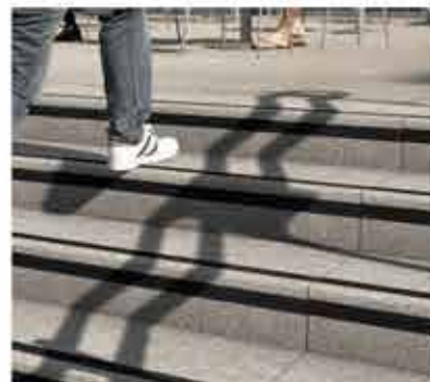
Concrete steps with natural aggregate
