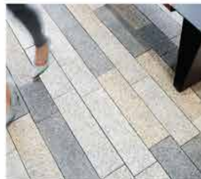
Feature concrete flag paving with natural stone aggregate
