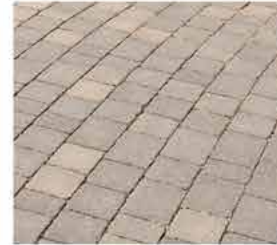
Tegula permeable concrete block paving
