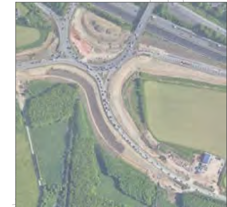
NORTH SOUTH AERIAL VIEW
