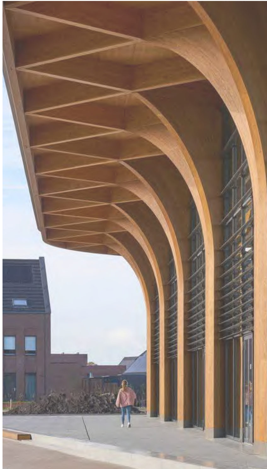
Sustainable Material - Exposed Glulam Structure
