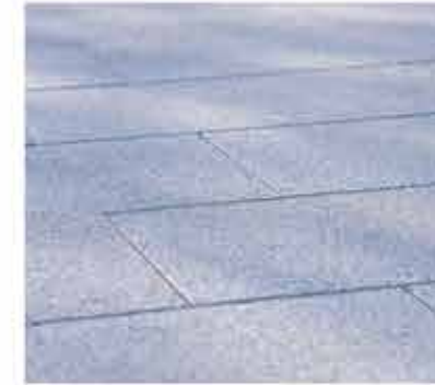
Concrete block / flag paving
