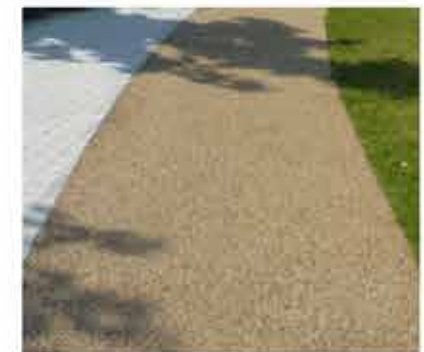
Resin-bound gravel feature paving
