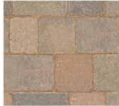
Tegula concrete block paving
