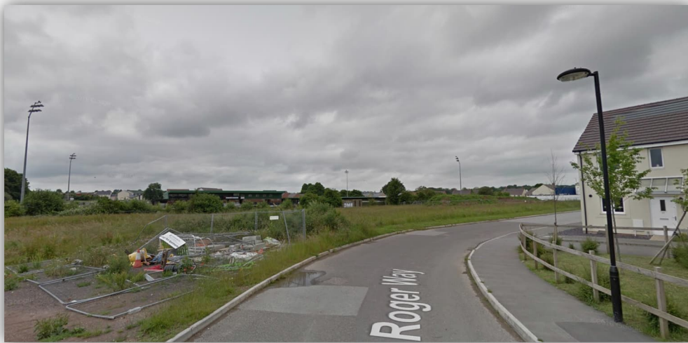
Figure 3.3: Existing street lighting columns
