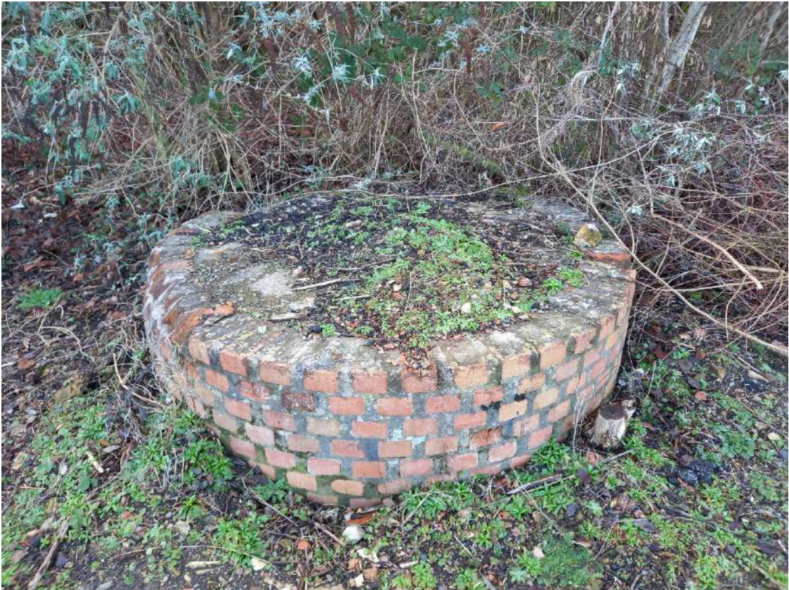
Image EDP A1.11: View of the airshaft within the site.
