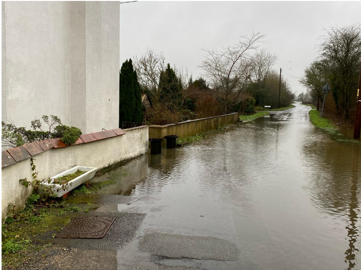
Outside 2 Chelworth Road, looking South West. Proposed cemetery entrance visible on the right.
