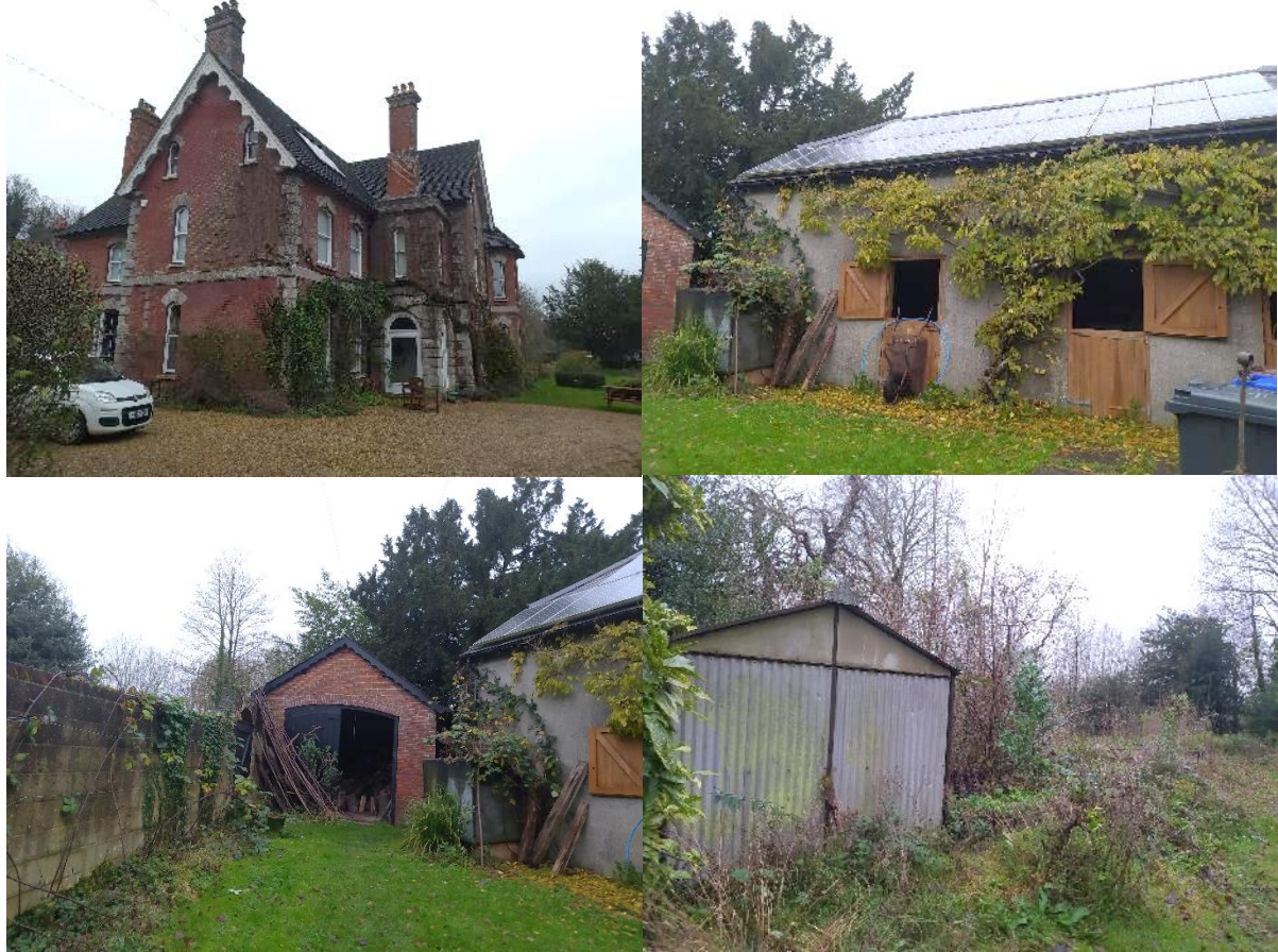
Figure 7. View of the buildings present on site (taken December 2023).
