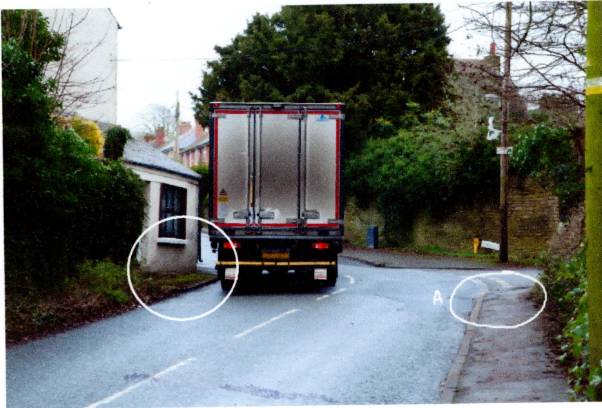
Fig A shows dip in kerbstone makes it easier for vehicle to mount pavement. On left hand side of vehicle, objects overhang pavement. Also no indication that pavement comes to an end when walking downhill outside 45 Marlborough Road.
