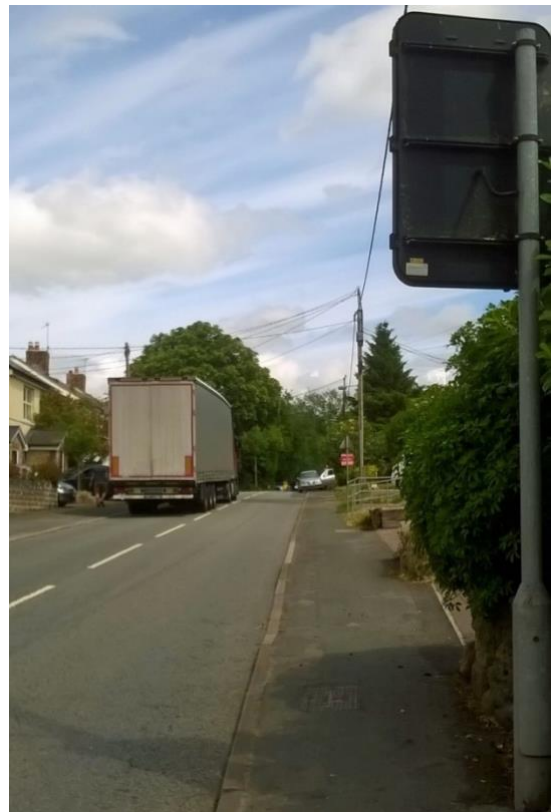
Below Right: Yet another example of LGV on unsuitable road
