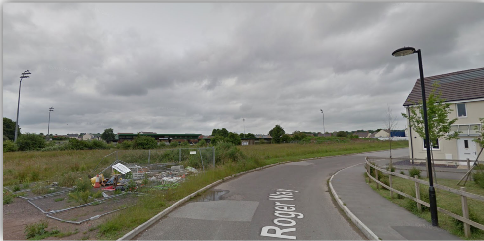
Figure 3.3: Existing street lighting columns
