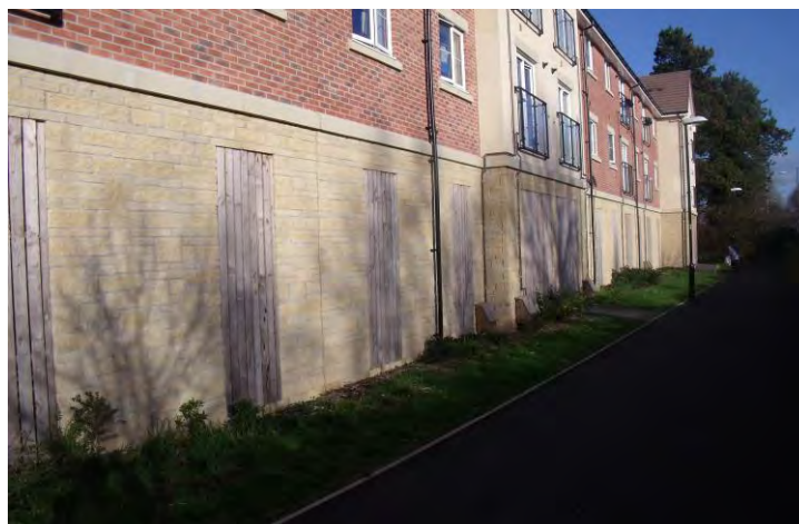
Photograph 2.3: The Vacant Ground Floor of Block C of the Local Centre, forming the site of Area G
