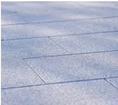
Concrete block / flag paving
