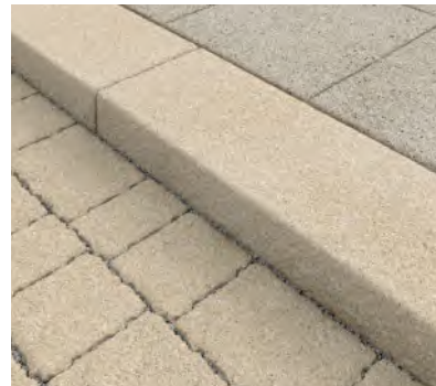
Concrete aggregate kerb in primary locations
