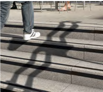
Concrete steps with natural aggregate
