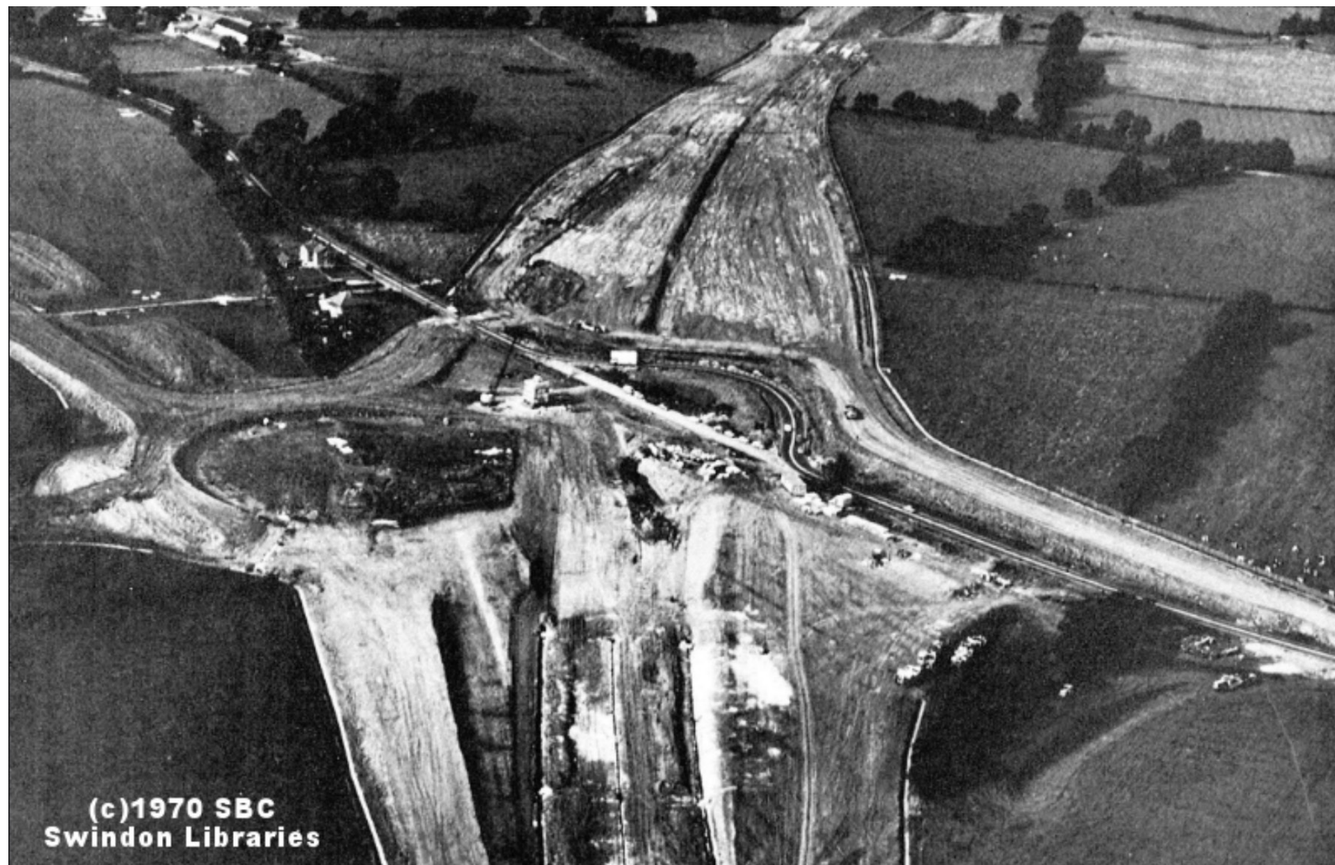
Figure 3.3 - Archive Photograph of construction of Junction 16, M4 Swindon, circa 1970.
