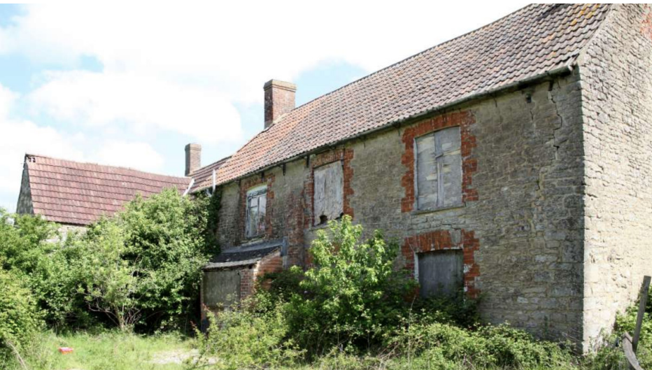
Figure 4.3. Studley Grange Farmhouse (source: Save Britain's Heritage).
