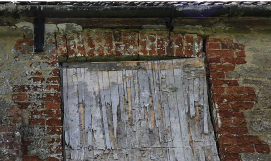
Figure 4.4. Studley Grange Farmhouse (source: Save Britain's Heritage).
