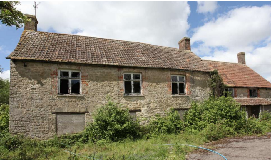
Figure 4.2. Studley Grange Farmhouse (source: Save Britain's Heritage).
