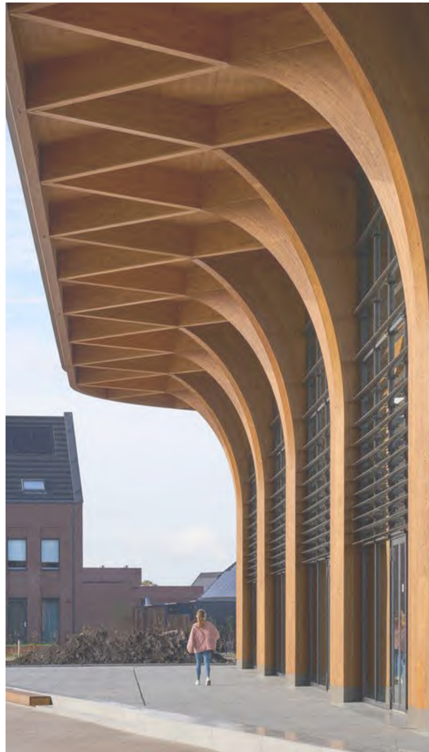
Sustainable Material - Exposed Glulam Structure
