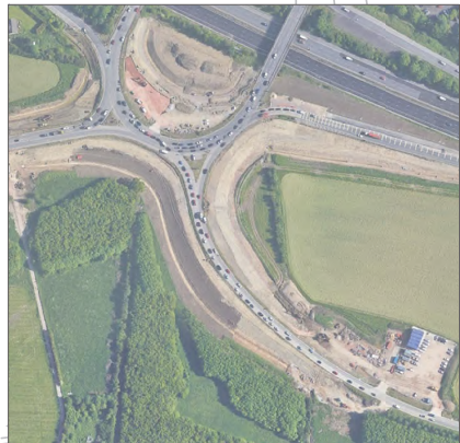
NORTH SOUTH AERIAL VIEW
