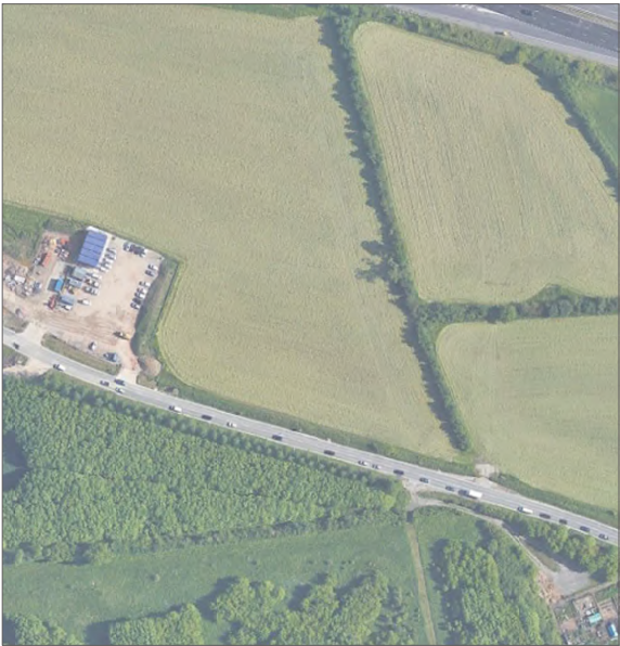
NORTH SOUTH AERIAL VIEW
