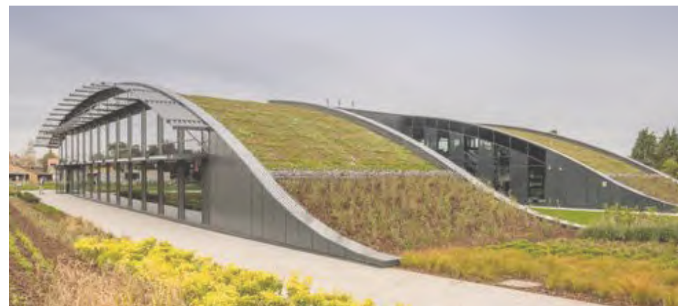
Roof - Sensible Architecture
