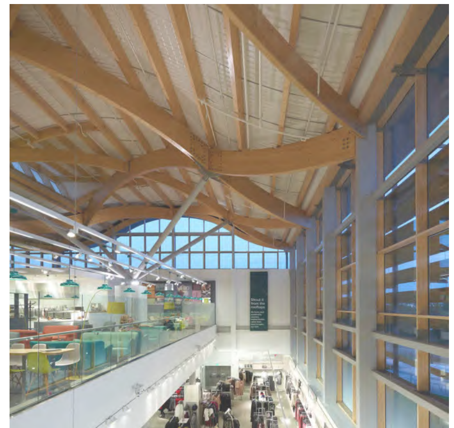
Sustainable Material - Exposed Glulam Structure
