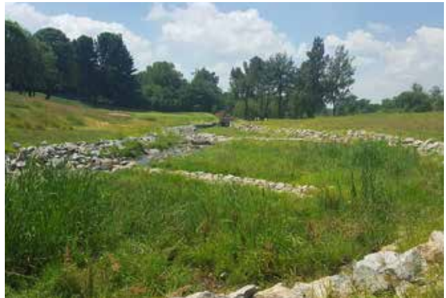
Dry attenuation basin
