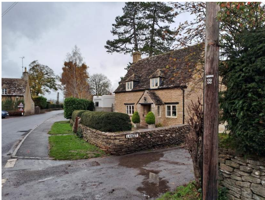
Plate 11 C18 Langet Cottage (1341007)
