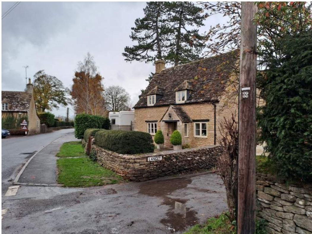
Plate 11 C18 Langet Cottage (1341007)
