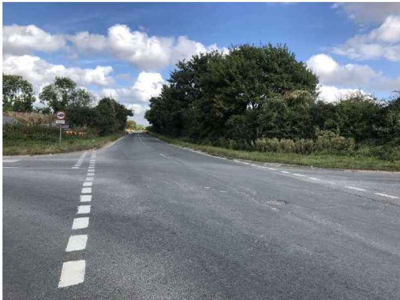
Figure 3-8 Ashton Road/Ewan Road Cross Road Junction – View North
