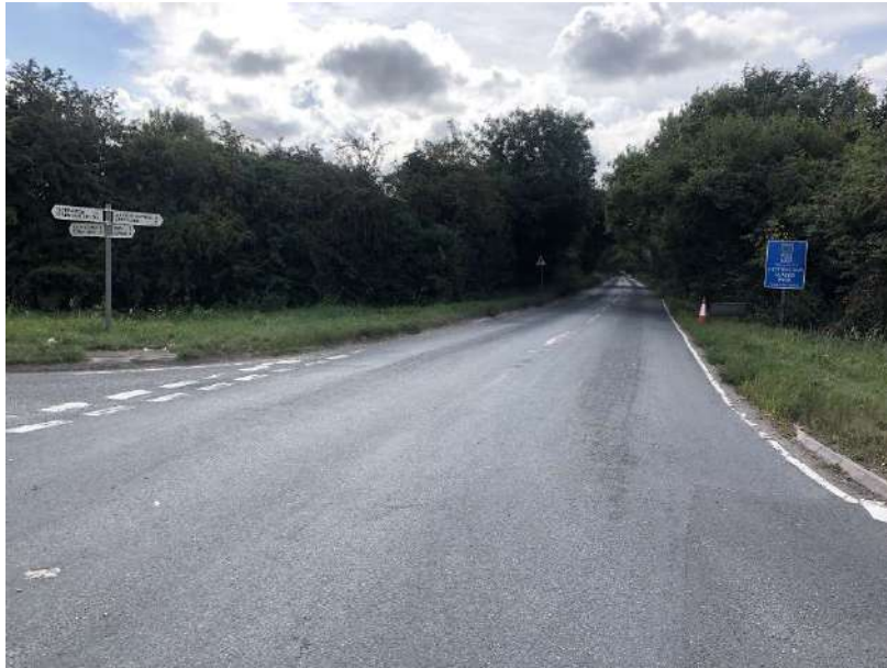
Figure 3-7 Ashton Road/Ewan Road Cross Road Junction – View South
