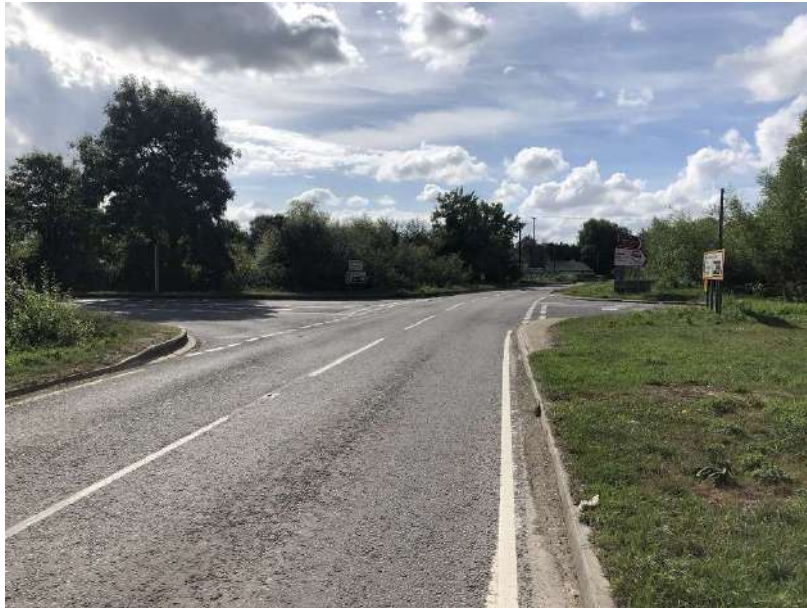
Figure 3-12 Ashton Road/Spine Road Cross Road Junction – View South
