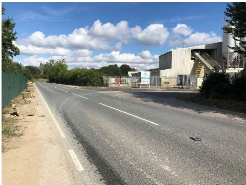
Figure 3-5 Aggregate Industries Site
