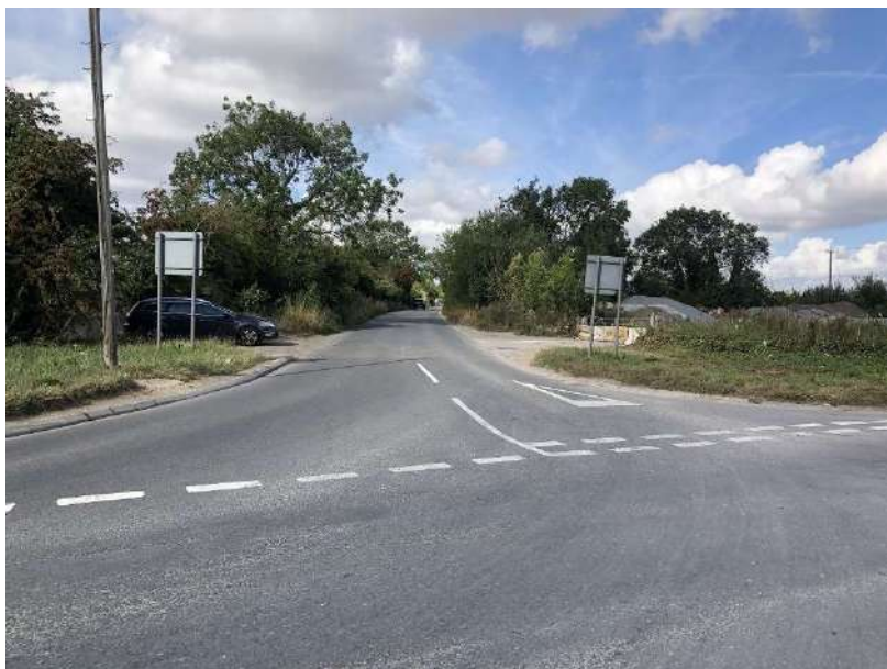
Figure 3-10 Ashton Road/Ewan Road Cross Road Junction – View West
