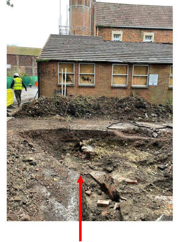
Original foundations of Mill House
