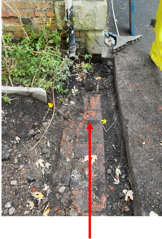
Original foundations of Mill House
