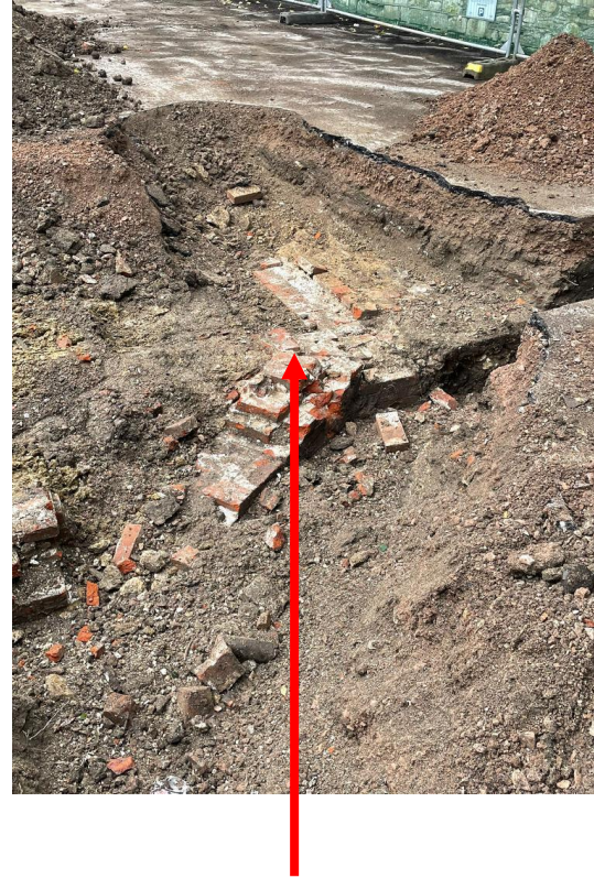
Original foundations of Mill House
